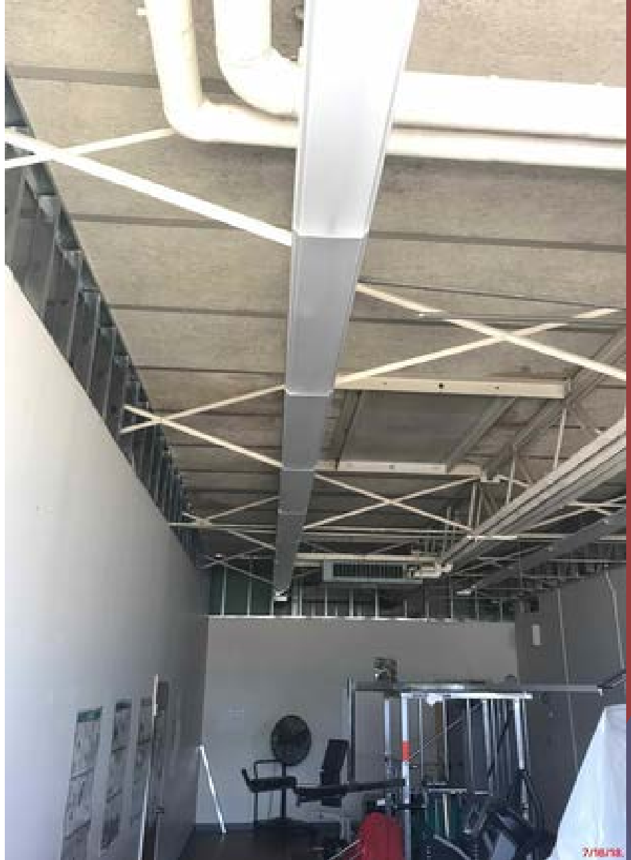
Patriot Org – Weigh/IT Rooms partition wall installation
