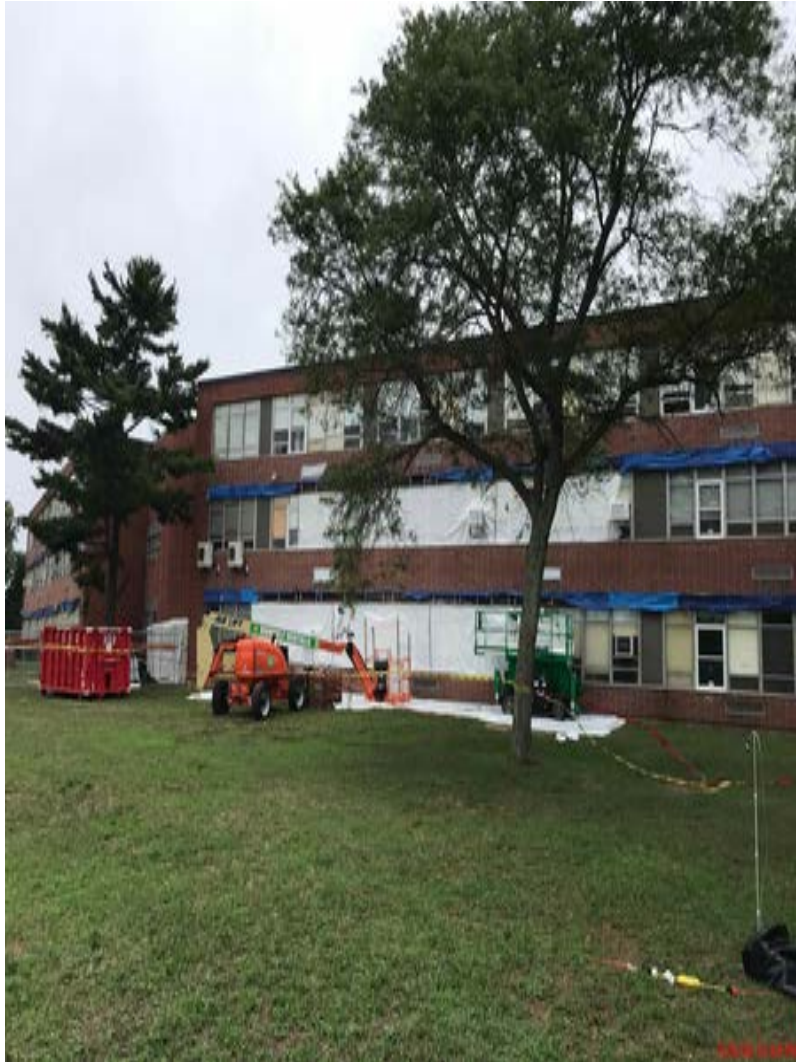
A1 Construction – East elevation flashing replacement
