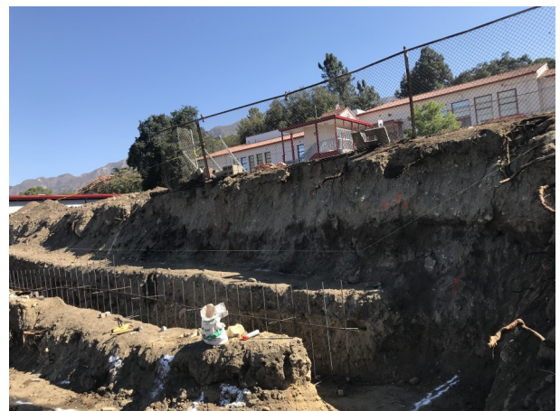
Monte Vista Elementary School New Building - Construction
