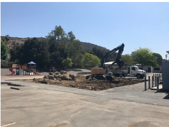
Glenoaks Elementary School New Building - Construction
