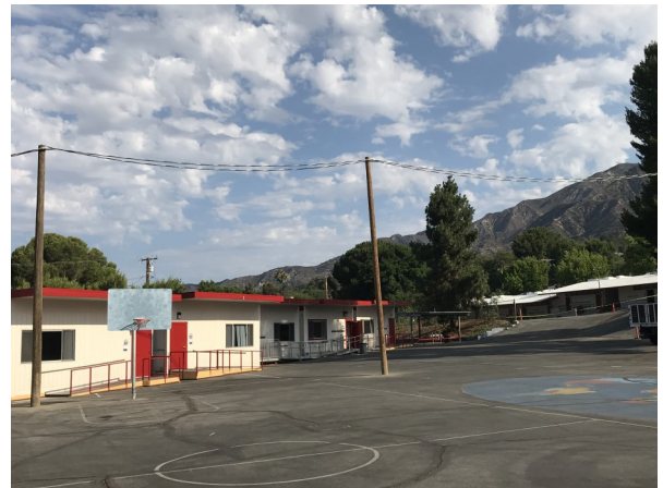
Monte Vista Elementary School New Building - Interim Housing
