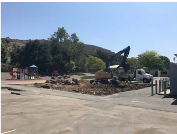
Glenoaks Elementary School New Building - Construction
