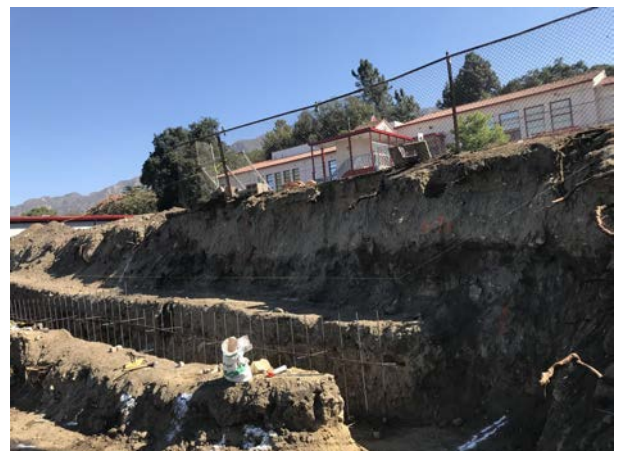
Monte Vista Elementary School New Building - Construction
