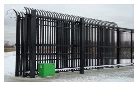
This would be our rolling gate design at 7 feet high with metal screening shown on the next picture of the Entry Gate below.
