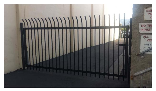
This would be the swing gate design for the north west wall with metal screen incorporated in the gate like the small entry gate at a height of 7 feet with two of this door designs at 15 feet each making a total of 30 feet.
