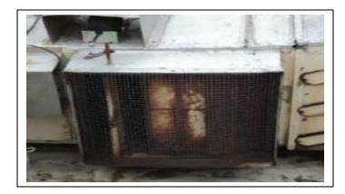
**Brief Description:** Replace deteriorated HVAC units in the 2000 & 3000 buildings. Install new HVAC Control
