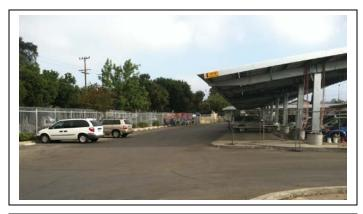
**Brief Description:** New 133.77kW Photovoltaic generating project. This project has 3 shade structures to be installed in the playfield area.
