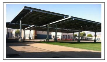
**Brief Description:** New 147.49kW Photovoltaic generating project. This project has 3 large and 2 minor shade structures to be installed in the playfield
