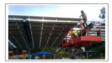
**Brief Description:** New 107.5 kW photovoltaic generating project. This project has 2 large shade structures located on playing field with direct student access.
