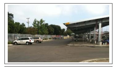
**Brief Description:** New 354.9 kW Photovoltaic generating project. This project has 4 carport structures and two large ground mounted systems
