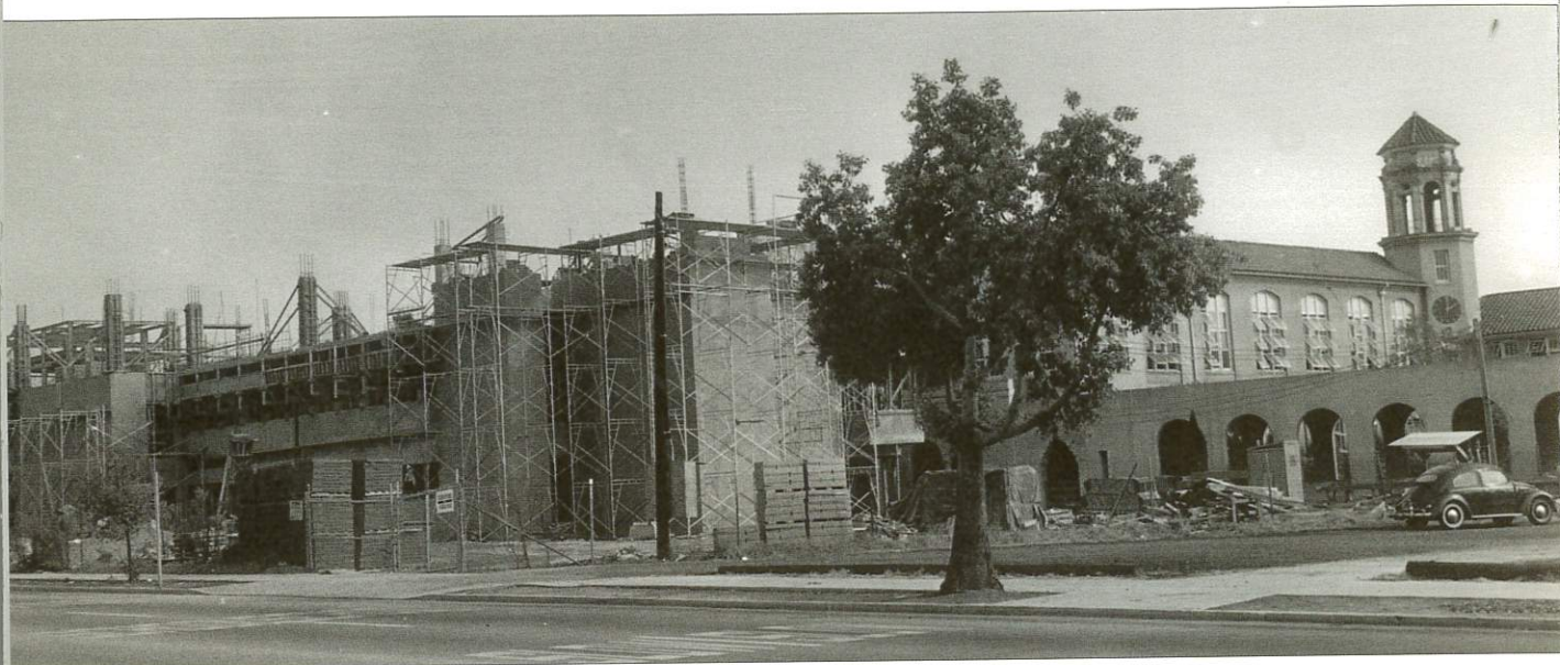
Current building on Broadway under construction with bell tower at right (circa 1967)
