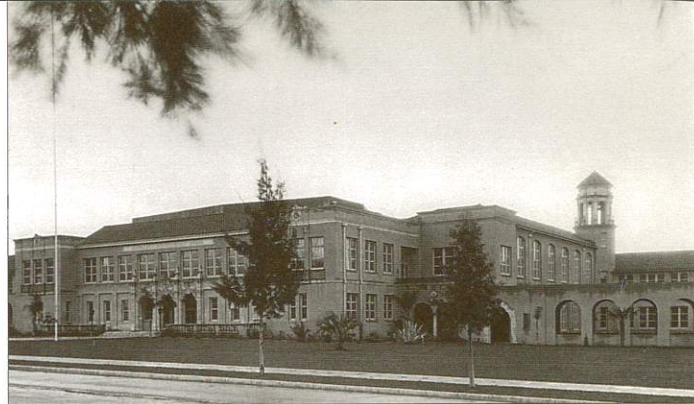
Entrance to the main building from Broadway; circa 1930s
