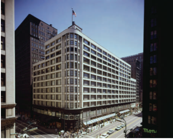
Carson, Pirie, Scott and Company Building © Hedrich Blessing Collection/Chicago History Museum/Getty Images
