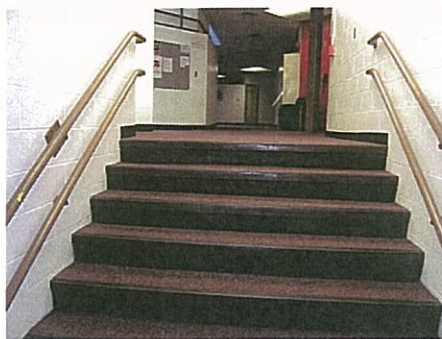
Stairs to upper level
