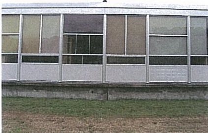
Typical storefront on north elevation
