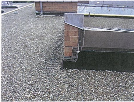
Flashing repairs supported and identified
