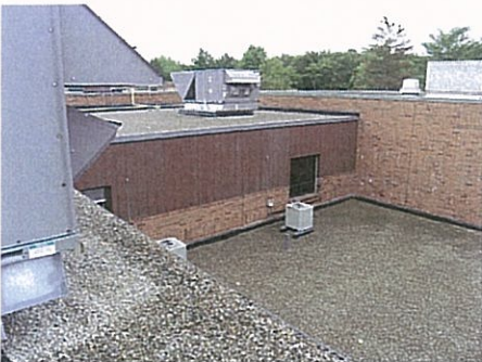
Lower roof areas in good condition
