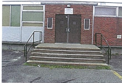
Service doors at east elevation
