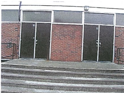
Exit doors at gymnasium
