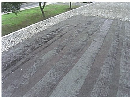
Repair areas along south side of building
