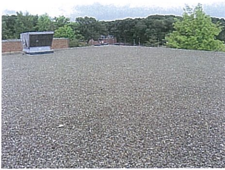
General condition of roofing
