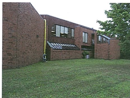
Sloped glazing at first-floor classrooms
