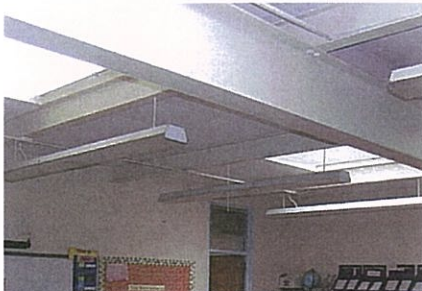
Typical steel framing at classroom
