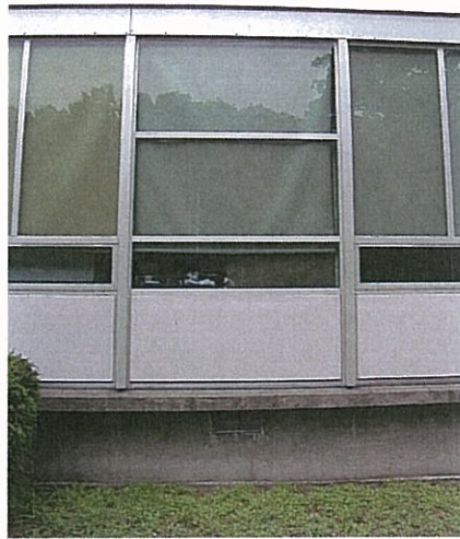
Storefront at core wing – south elevation
