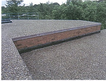
Flashing in good condition; fall protection in place at roof edge.
