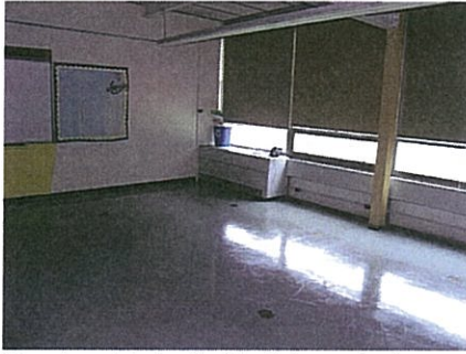
View from interior (cafeteria/gym wing)
