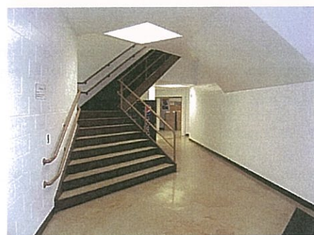
Typical stair finishes
