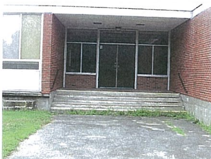
Typical exit doors at north elevation
