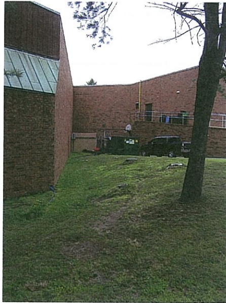
Pool water pumped and daylighted at grade
