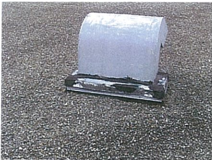
Hood flashing repaired with mastic
