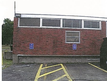
Clerestory windows on east elevation (Lower window is a later renovation)
