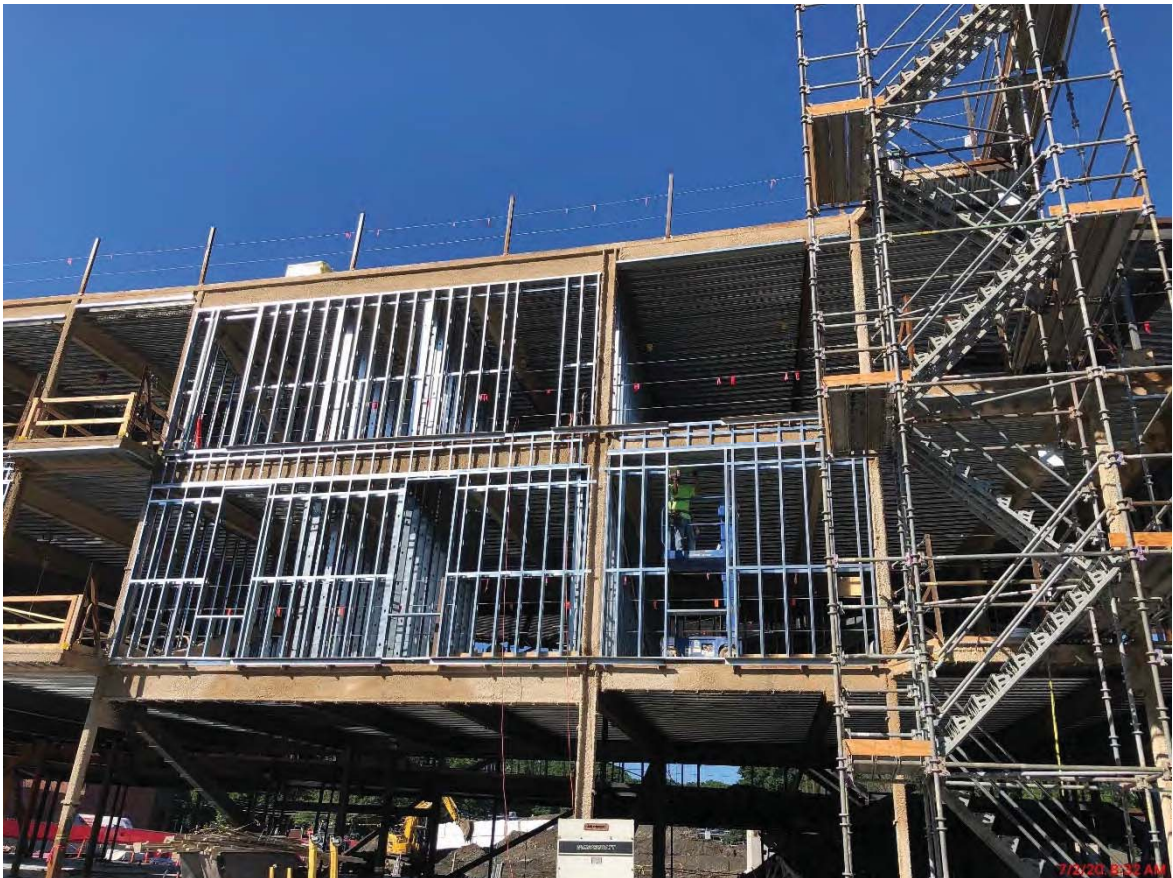
Photo 4: Exterior Framing has begun for the building envelope.
