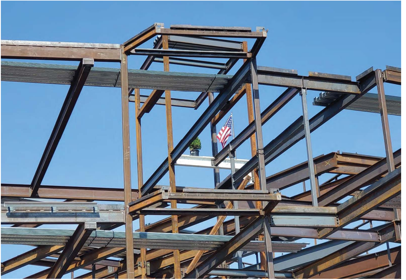
Photo 7: Topping-Off beam in it's final location
