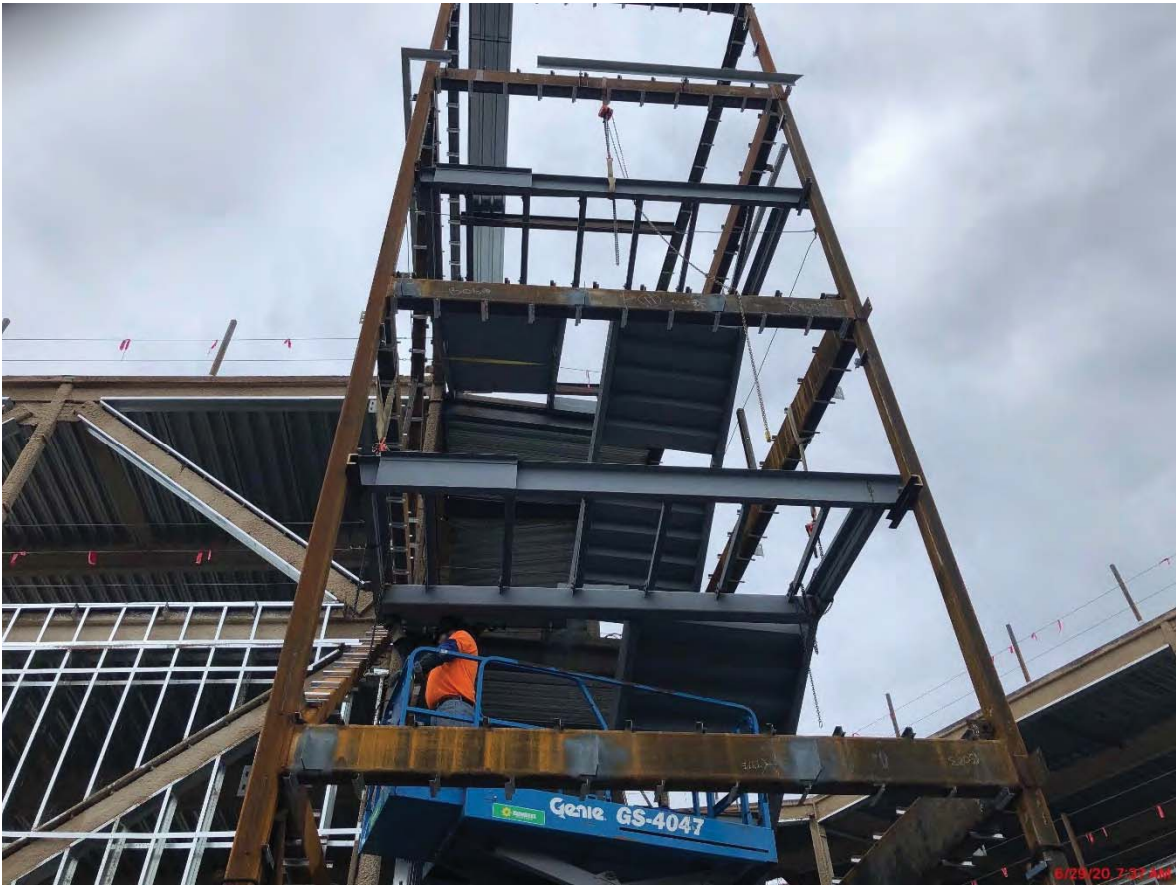
Photo 3: Stair 1 Erection (East Side of Building Area B) in progress
