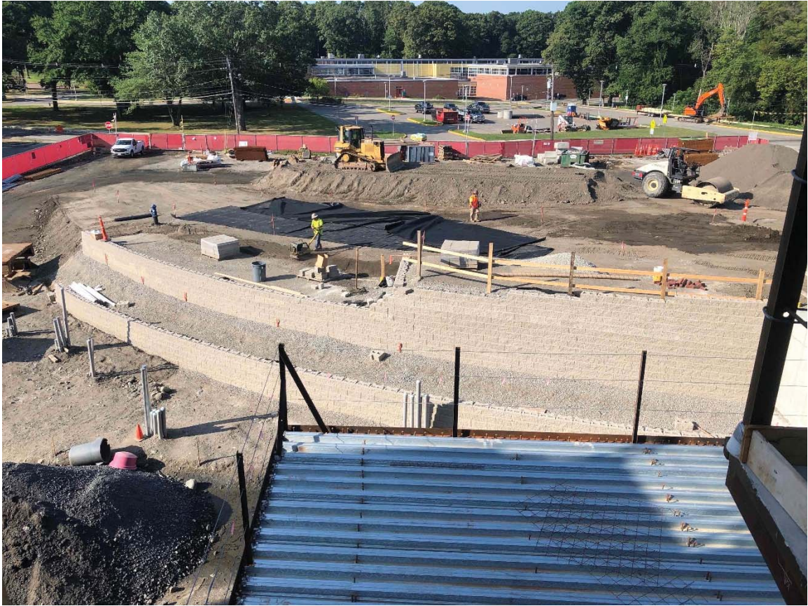
Photo 4: Eastern Retaining Wall nearing completion
