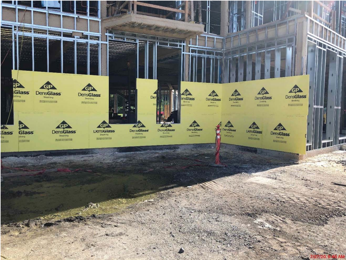
Photo 3: Exterior Sheathing has begun on South Side of Classroom Building
