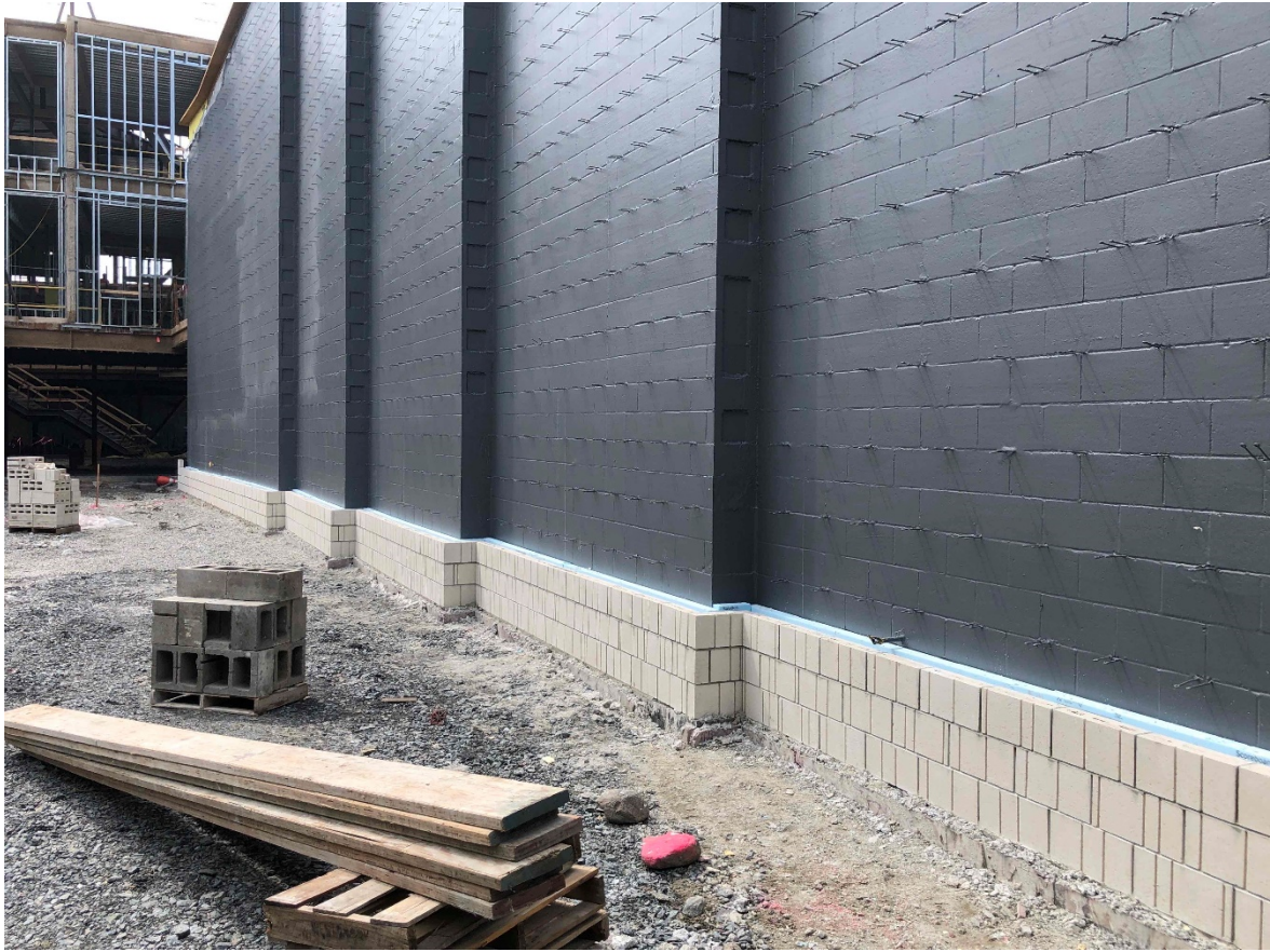
Photo 3: Masonry Façade work has begun on the gym and auditorium
