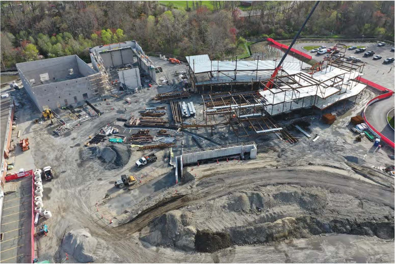
Photos 1 & 2: Aerial Drone Views of the site showing the steel/masonry building superstructure.
