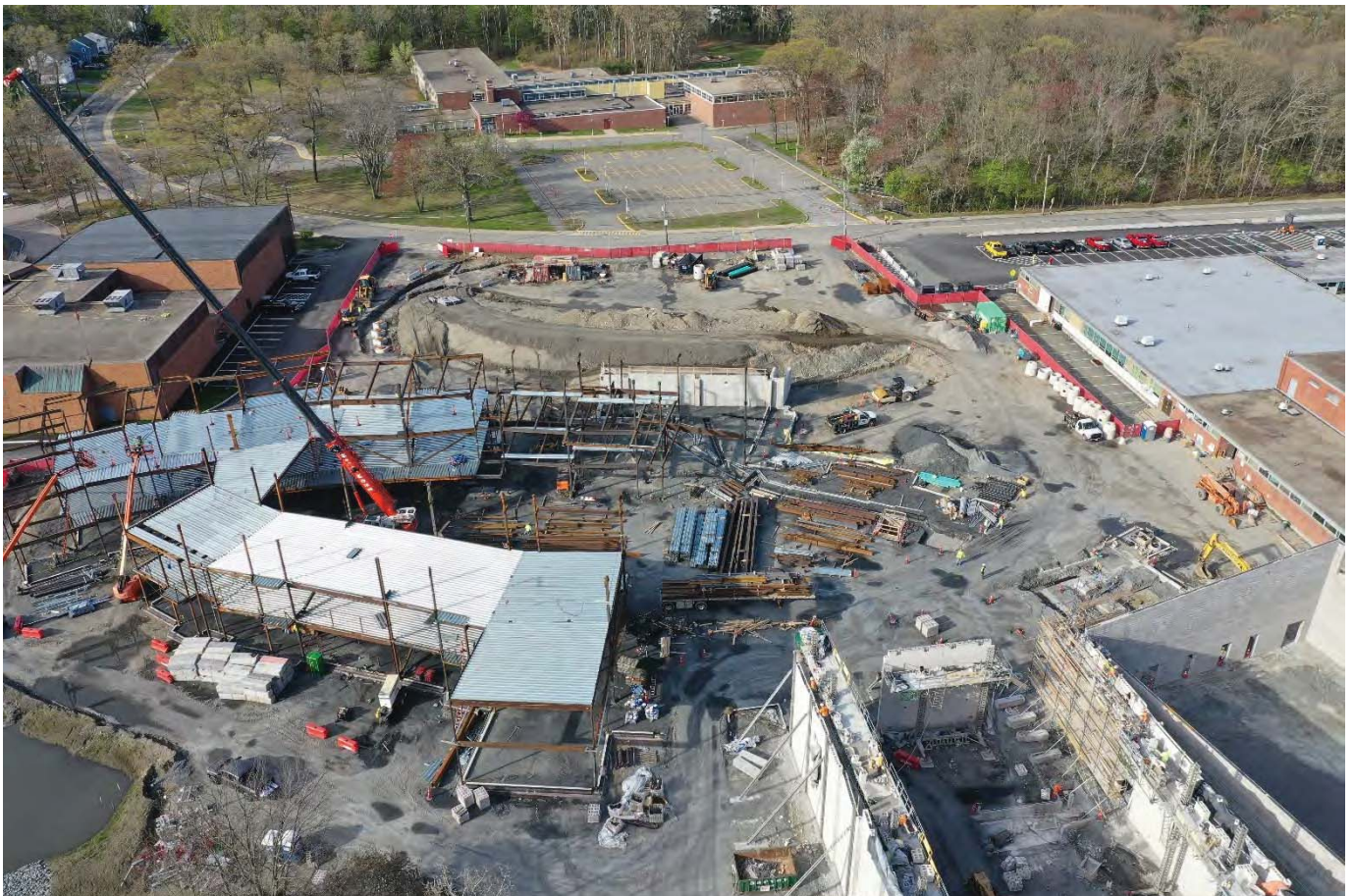
Photos 1 & 2: Aerial Drone Views of the site showing the steel/masonry building superstructure.
