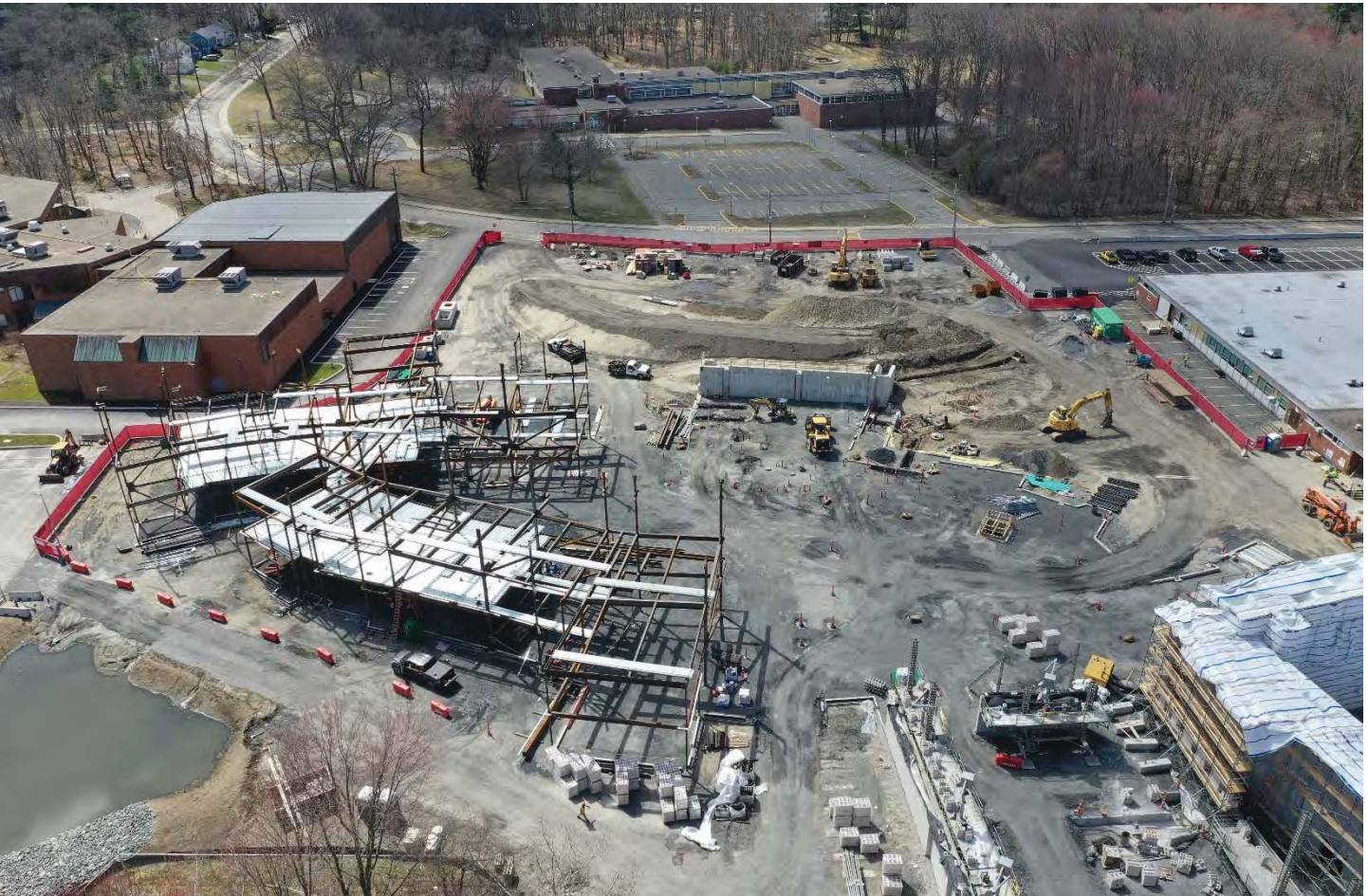
Photos 1 & 2: Aerial Drone Views of the site showing the masonry scaffolding enclosure for the gymnasium.
