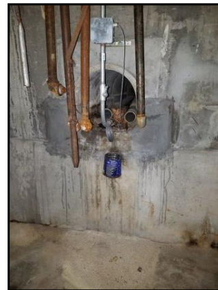
Abandoned Pipes (connection to former UST)
