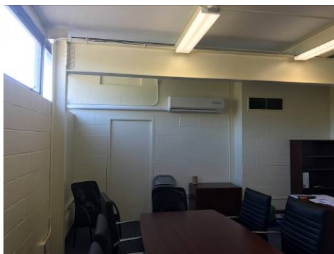
Community Health – Ductless AC Unit and Associated Roof Condensing Units
