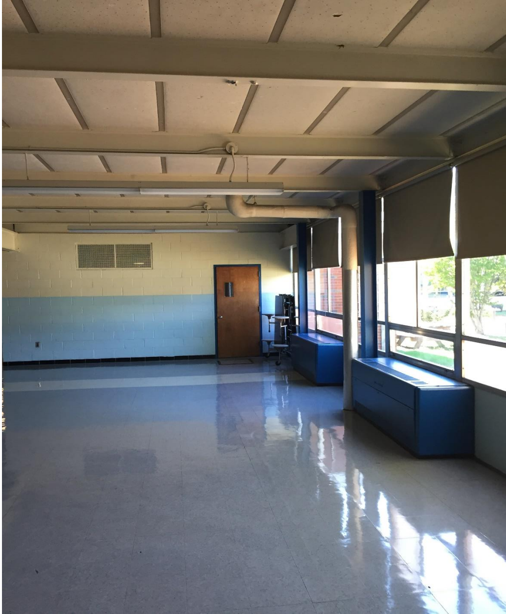
Roof Drain with ACM Fittings
