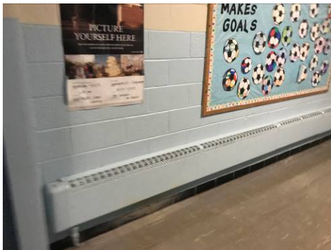
Corridor – Fin Tube Radiation Heating
