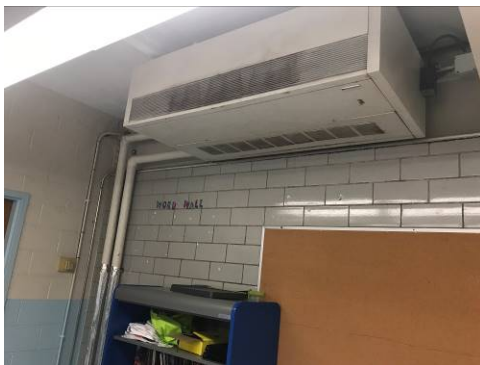
Horizontal Classroom Unit Ventilators
