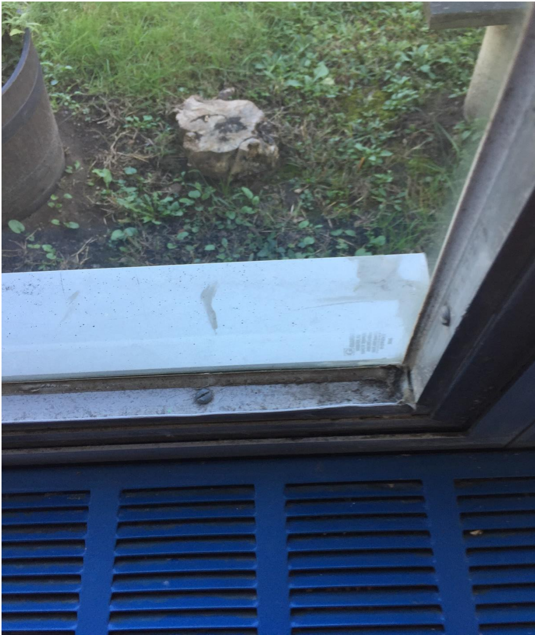
ACM Window Glaze, Interior Side of Exterior Window
