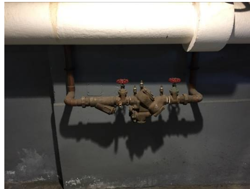
HVAC Equipment Make-Up
