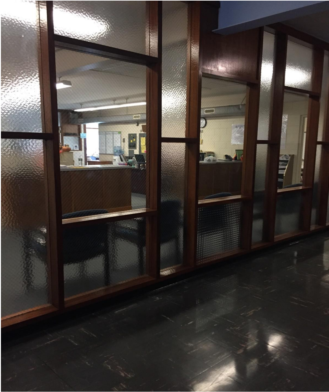
Interior ACM Window Glaze Associated with Wood Framed Windows
