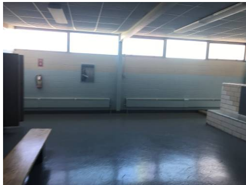
Typical Locker Room Fintube
