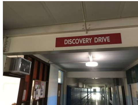
Office with Window AC installed in Interior Wall
