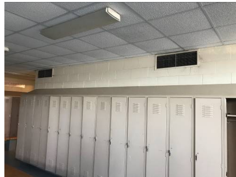
Typical Locker Room Exhaust
