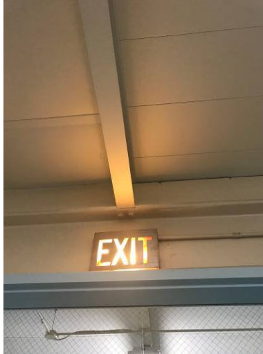
Old Functional Exit
