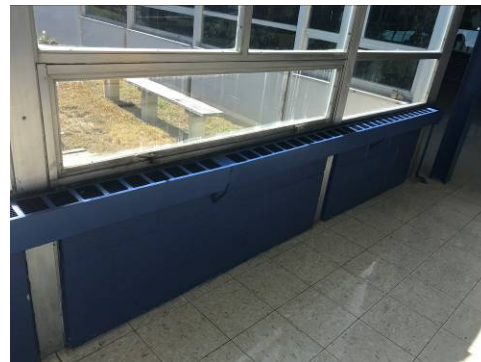
Corridor – Fin Tube Radiation Heating
