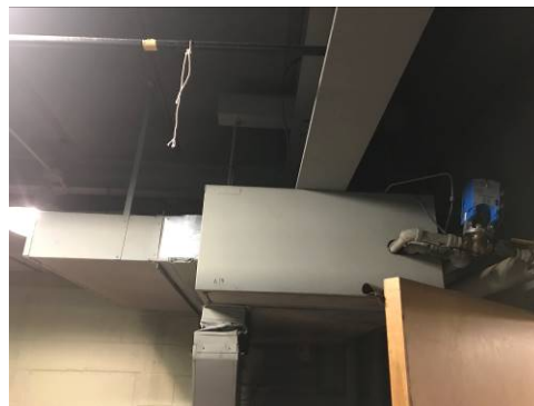
Horizontal Classroom Unit Ventilators
