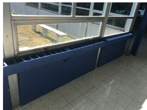
Corridor – Fin Tube Radiation Heating
