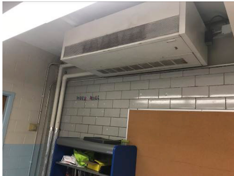
Horizontal Classroom Unit Ventilators
