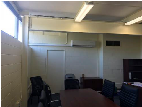
Community Health – Ductless AC Unit and Associated Roof Condensing Units
