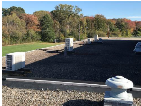
Community Health – Ductless AC Unit and Associated Roof Condensing Units
