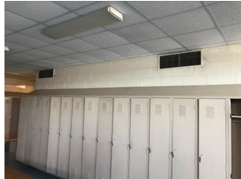
Typical Locker Room Exhaust
