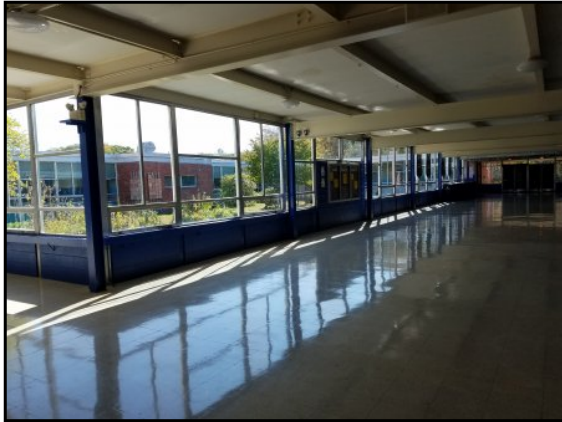
Typical hallway & view of courtyard
