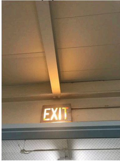
Old Functional Exit
