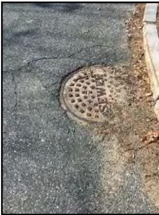
Storm drains in MBCC parking lot
