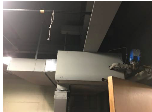
Horizontal Classroom Unit Ventilators
