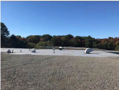
Roof – Exhaust Fans and Intake/Relief Hoods
