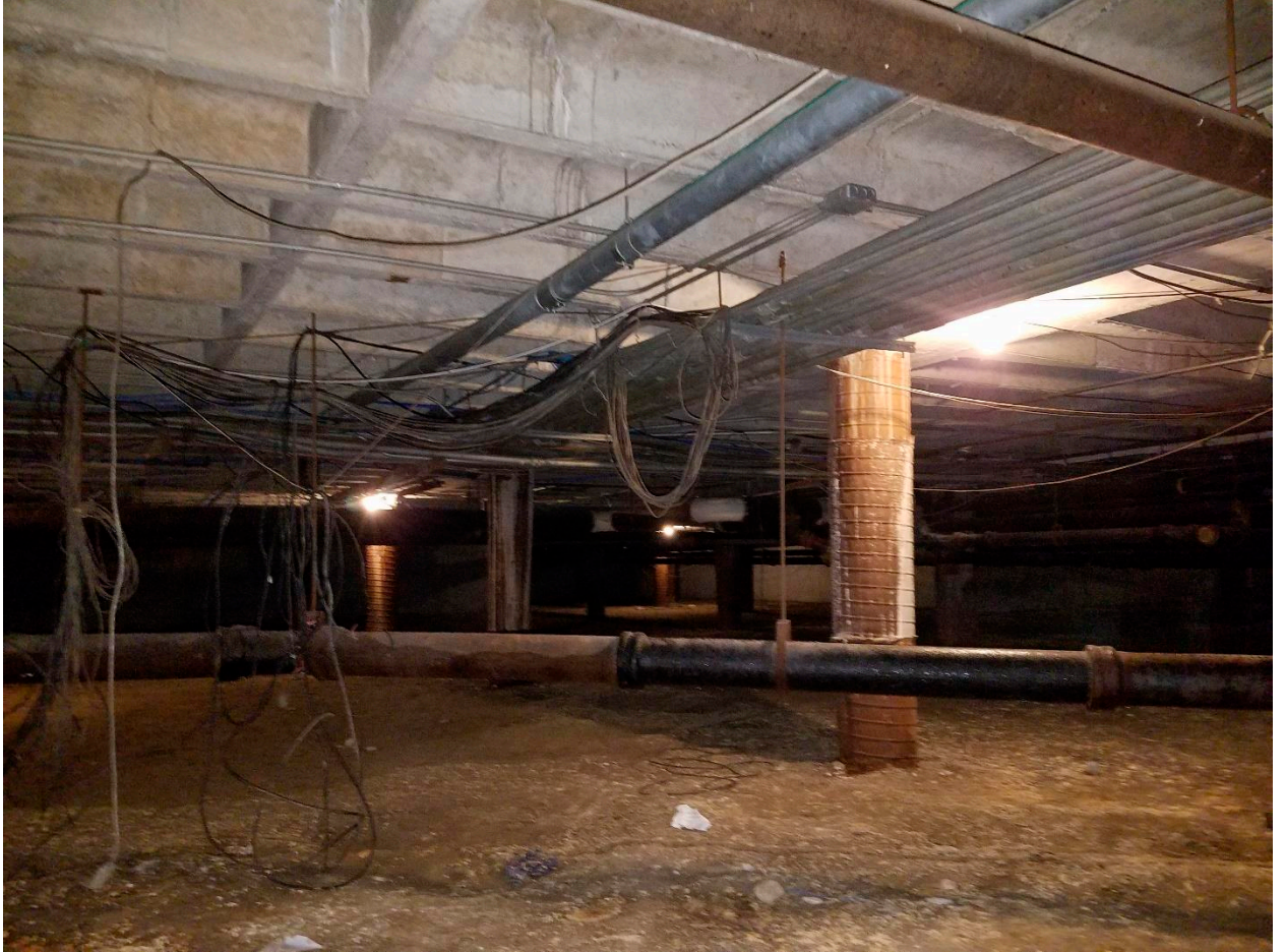
Crawl space area.
