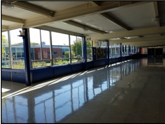
Typical hallway & view of courtyard
