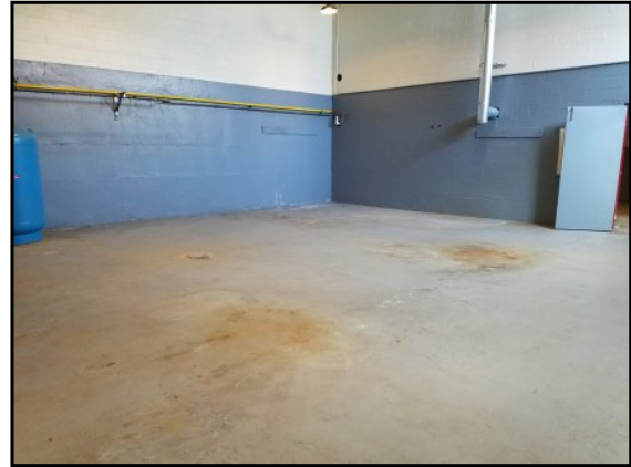
Boiler Room (basement level)
