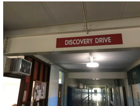
Office with Window AC installed in Interior Wall
