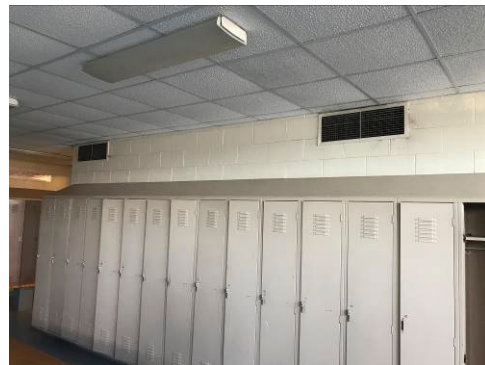
Typical Locker Room Exhaust
