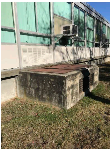
Entryway to Vault
