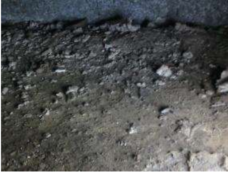
Pre-Cleaning H & V Supply Ductwork
