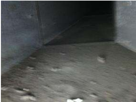
Pre-Cleaning H & V Supply Ductwork
