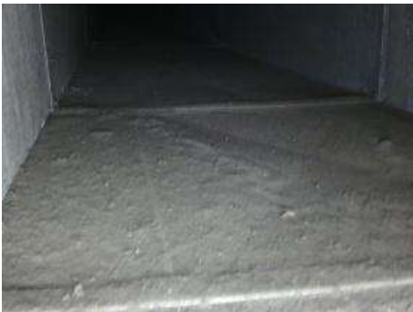
Pre-Cleaning H & V Supply Ductwork
