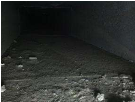
Pre-Cleaning H & V Supply Ductwork
