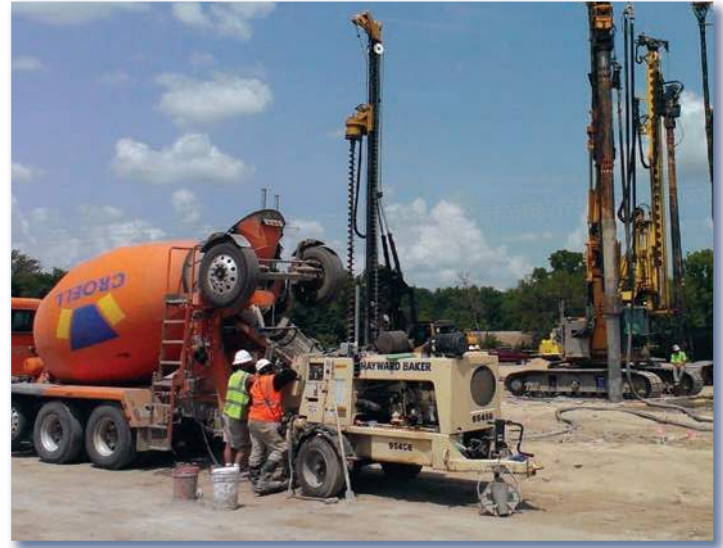
Pump transfers grout to RI tool.
