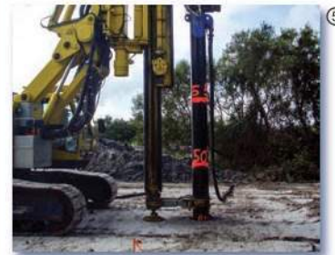
elevation. RIs reduced the schedule compared to surcharging and waiting for consolidation to occur.
