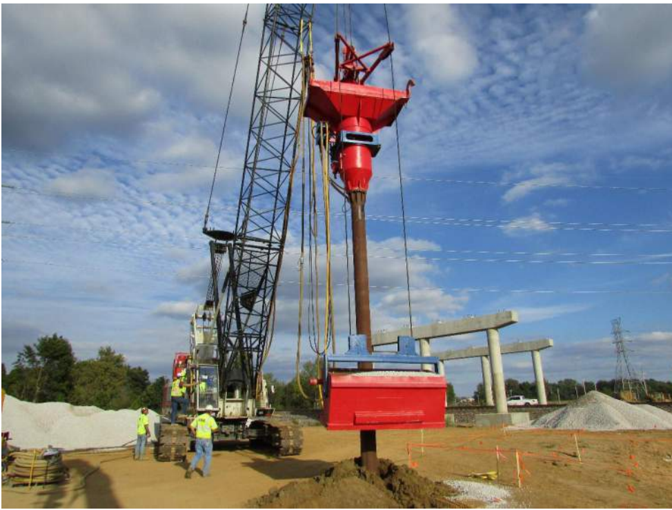
Fig 3 Installation of VSCs (dry bottom feed method) and of CMC rigid Inclusions (displacement auger)
