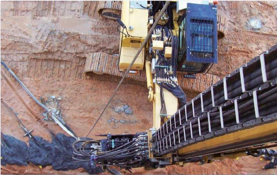
Rigid Inclusion installation for a planned hotel.
