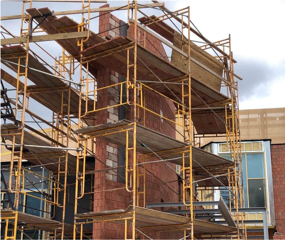
Photo 5: Chimney Section taking final shape
