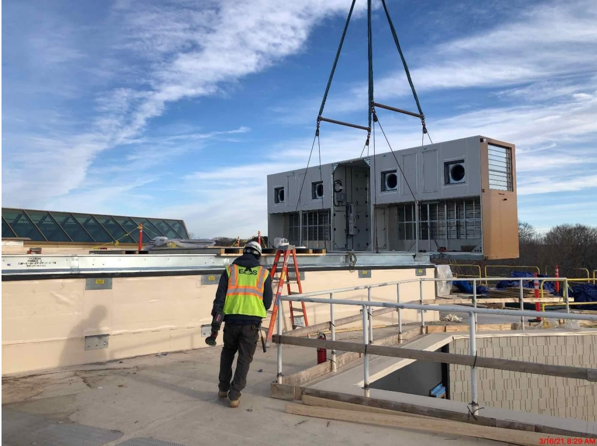
Photos 3 and 4: Chiller and RTU section being swung and set on the roof
