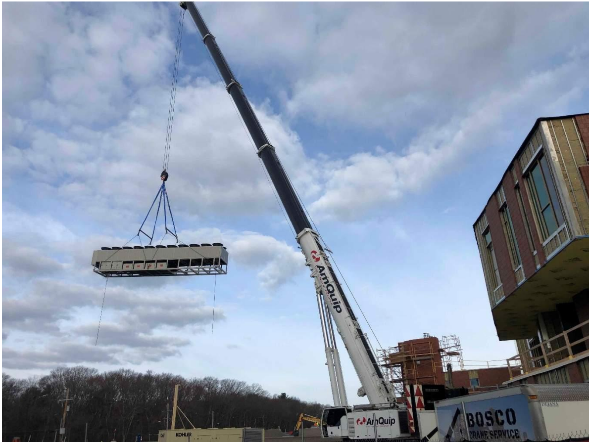
Photos 3 and 4: Chiller and RTU section being swung and set on the roof
