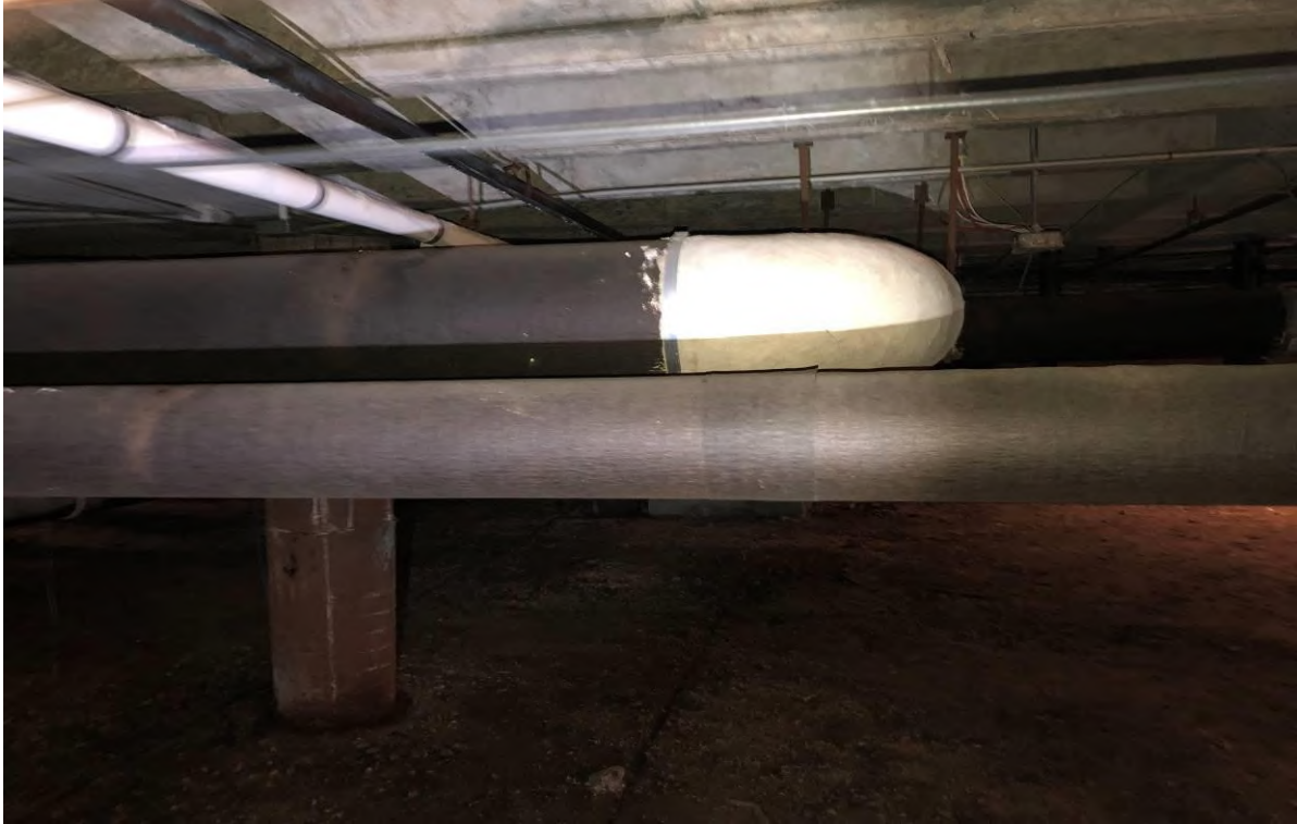
ACM Pipe Insulation in Crawlspace
