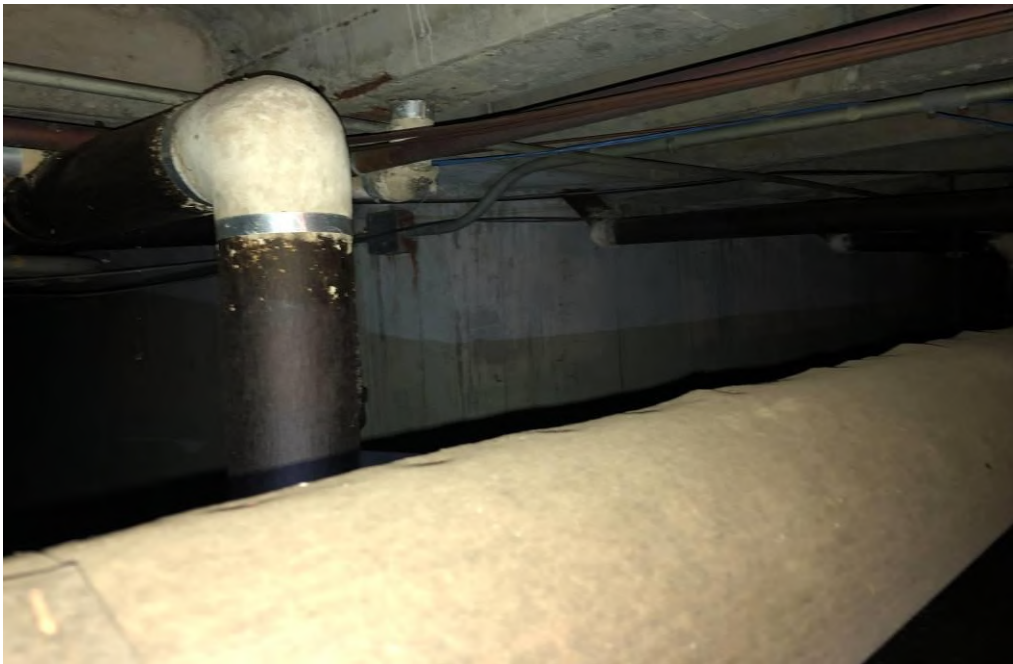
Typical ACM Pipe Fitting
