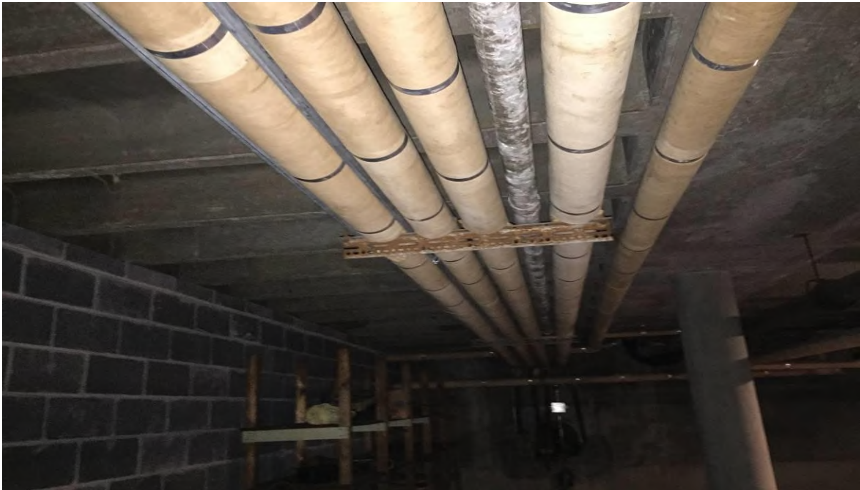
ACM Pipe Insulation in Crawlspace
