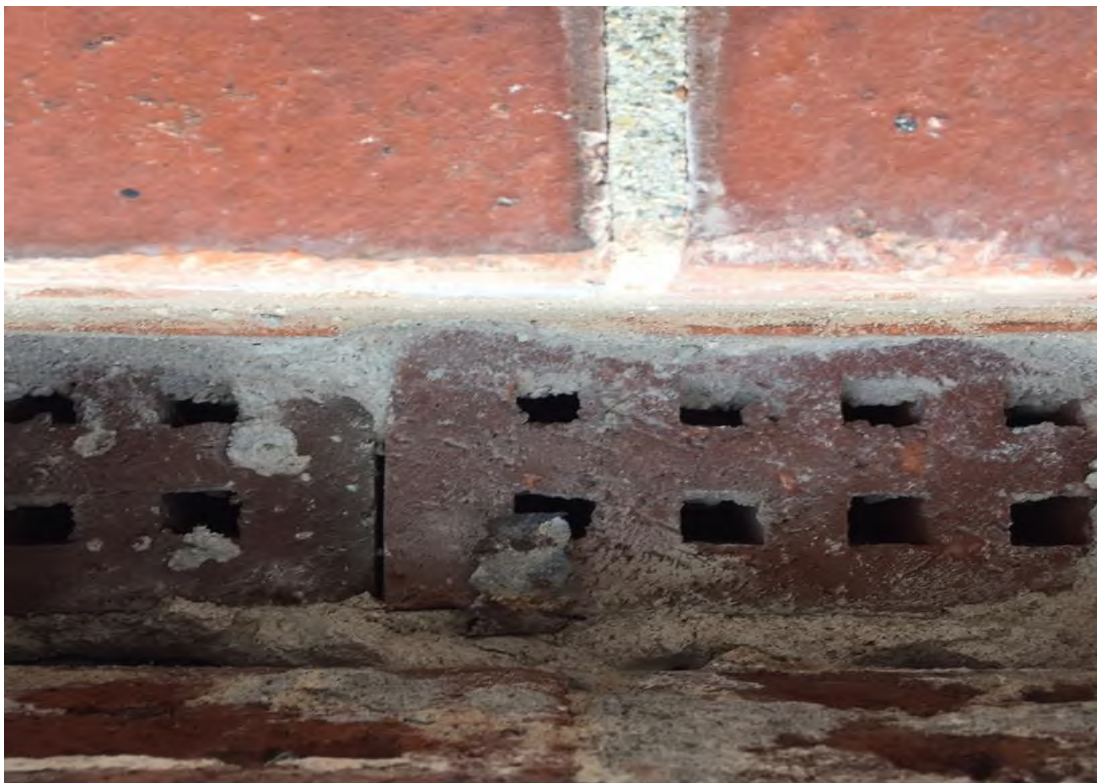
View Behind Brick Facade
