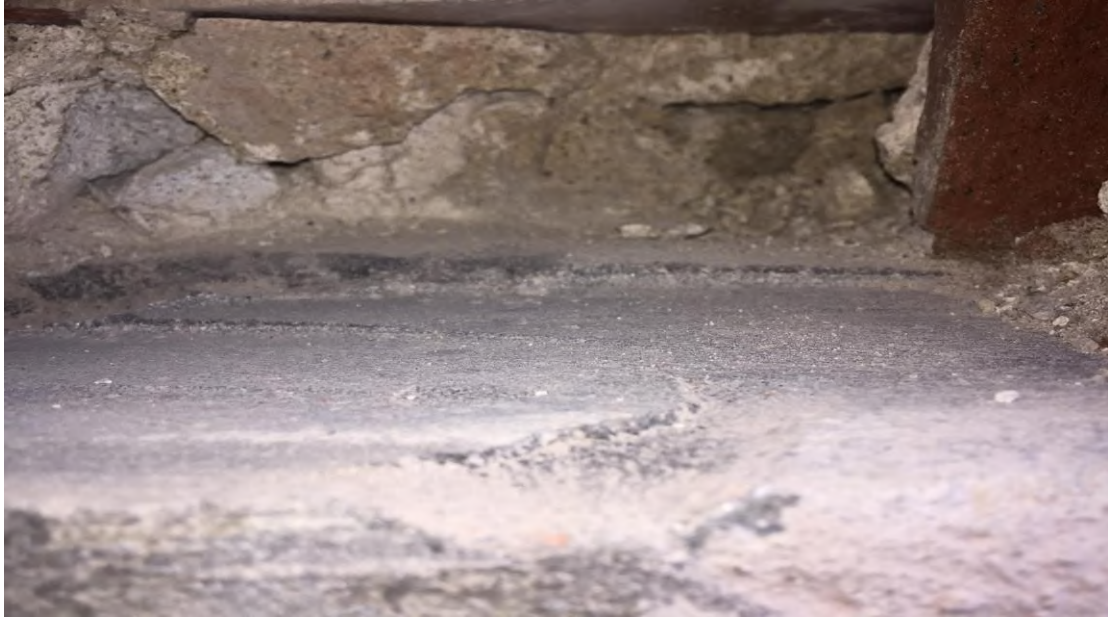
View Behind Brick Facade
