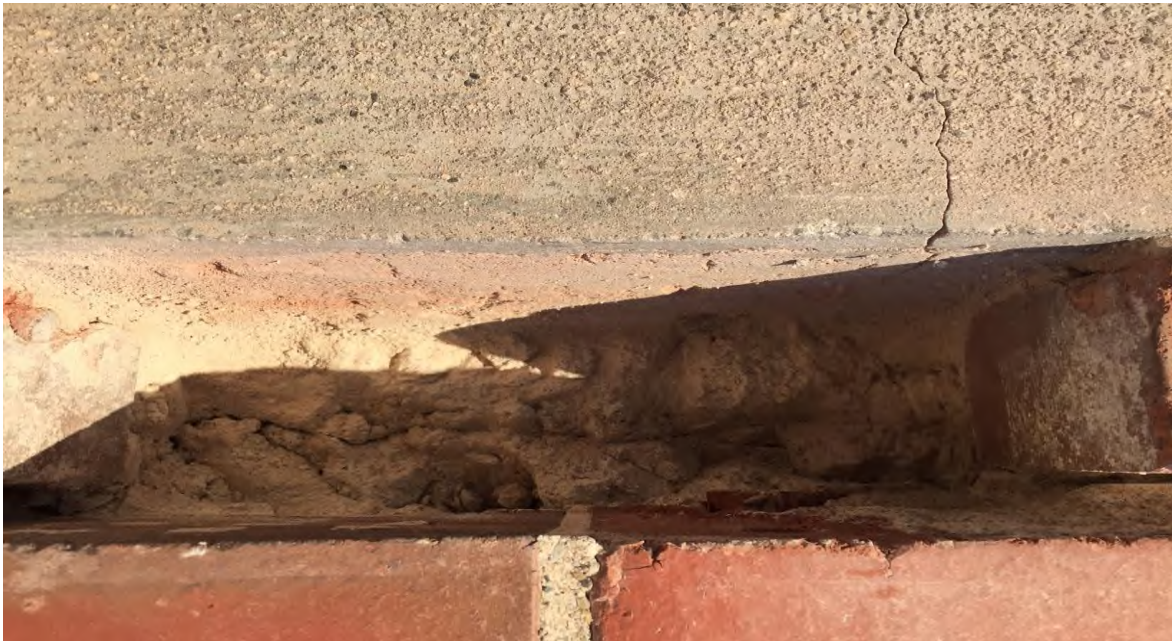
View Behind Brick Façade
