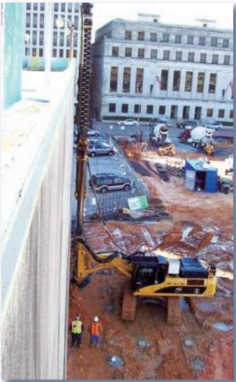
Above: HBI installed Rigid Inclusions on a congested downtown site for a hotel constructed on shallow spread footings.
