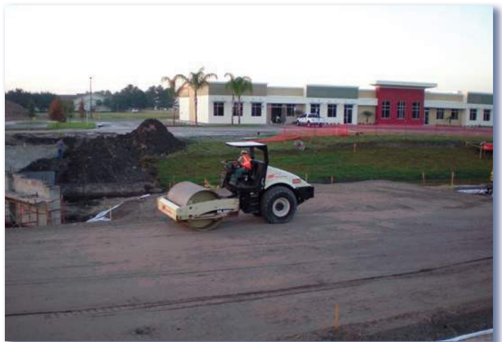
Compaction of granular structural fill during construction of an LTP for a slab supported by RIs.
