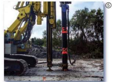
elevation. RIs reduced the schedule compared to surcharging and waiting for consolidation to occur.
