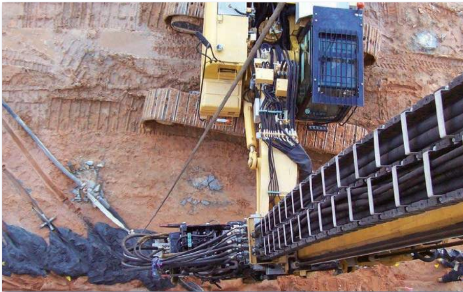
Rigid Inclusion installation for a planned hotel.
