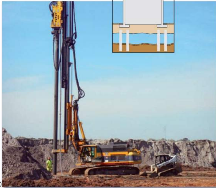
① RIs to support future fill and building loads for a grocery store.
