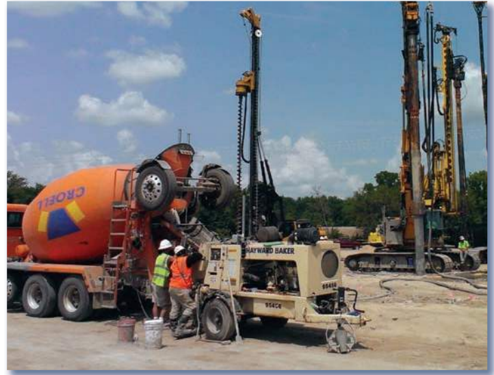
Pump transfers grout to RI tool.
