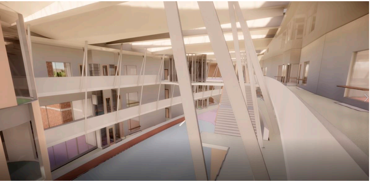
View of corridor balconies with structural tension straps, communicating stairs, and Breakout areas
