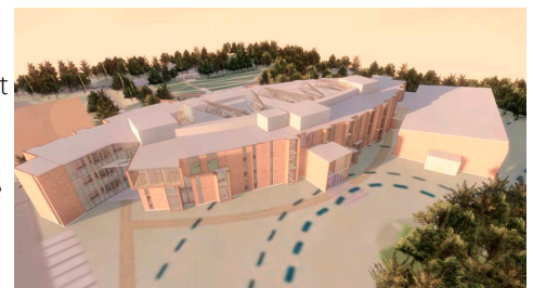
3-D model of massing, showing the two segmented arcs of classrooms and the Gymnasium/Auditorium.
