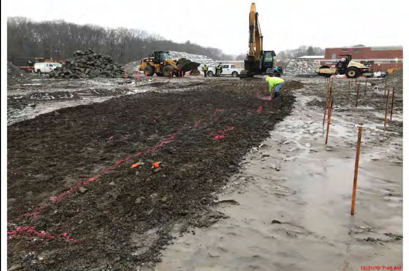
Photo 4: Remaining foundation excavation being laid out for Area "B".
