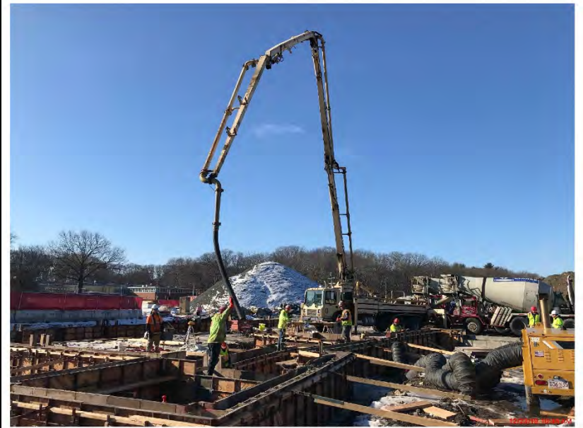
Photo 3: Concrete Pump staged at a stairwell foundation in Building Area "B"
