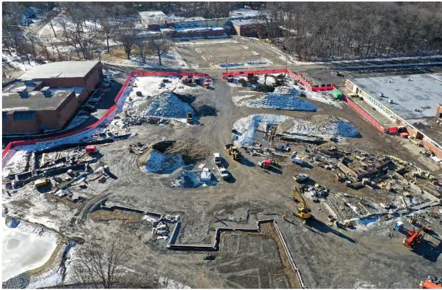
Photos 1 & 2: Aerial Drone Views of the site foundation footing progress.
