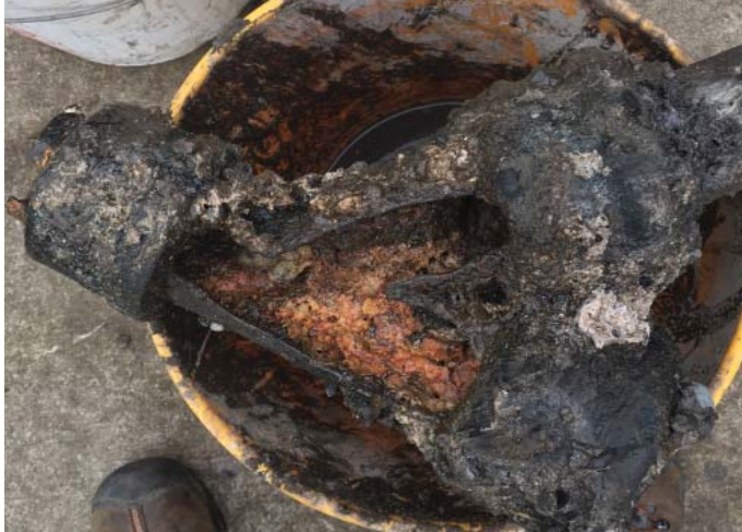
Camas Ridge Elementary School: Sewer Pipe
