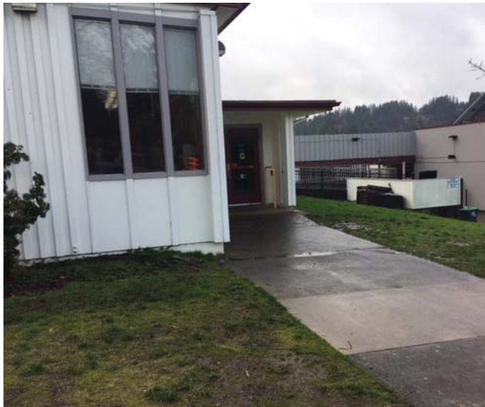
Adams Elementary: Unsecured Entry
