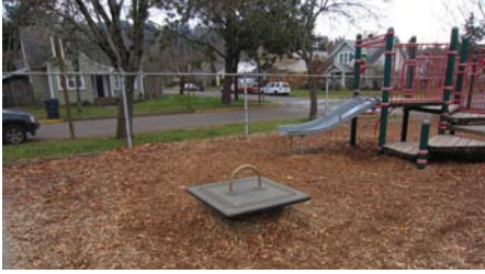
Fence surrounding outdoor play area does not have a turned top to prevent unauthorized entry
