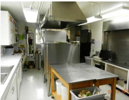
Existing kitchen is severely undersized
