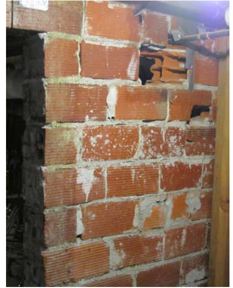
Existing hollow clay tile walls in the crawl space
