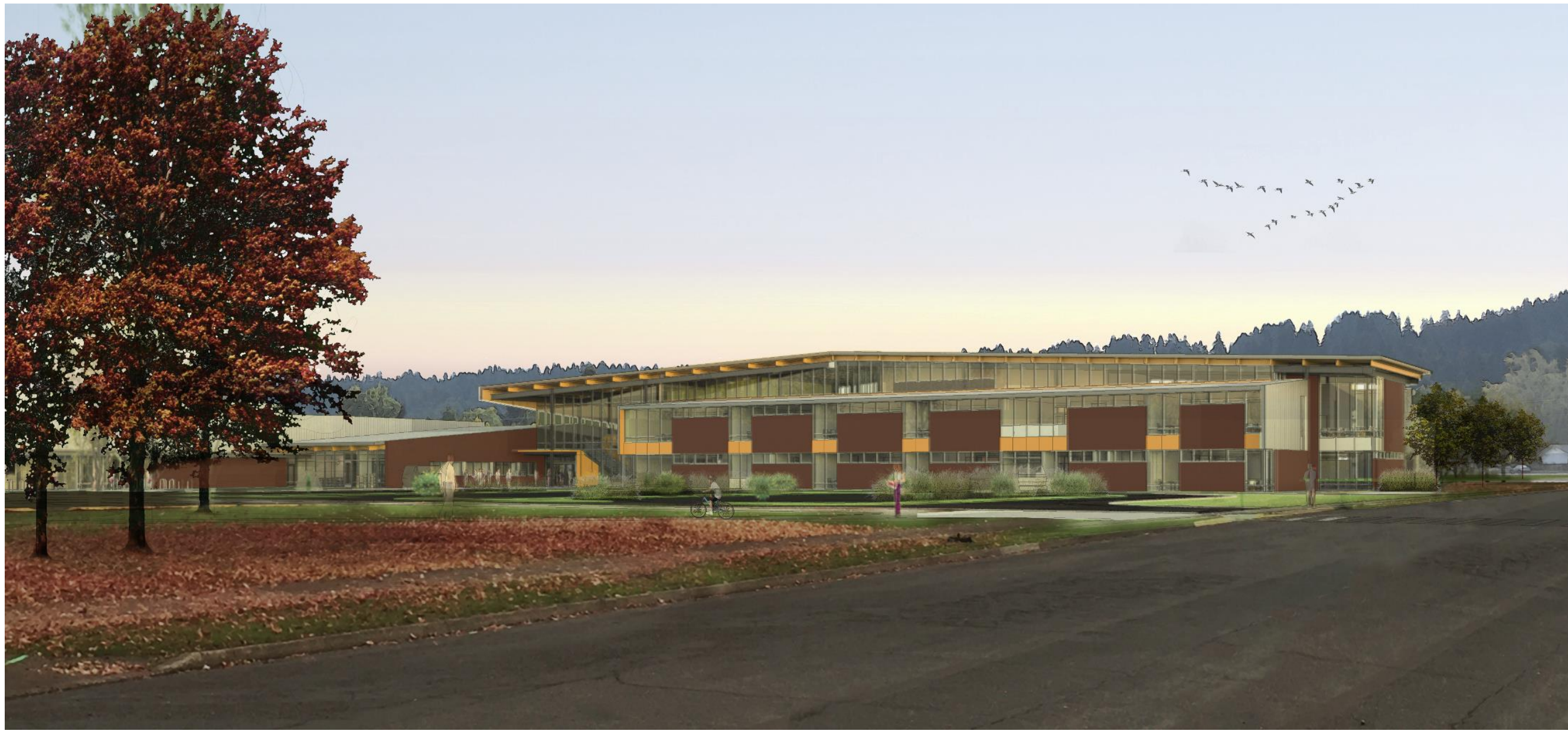
VIEW FROM NORTH
