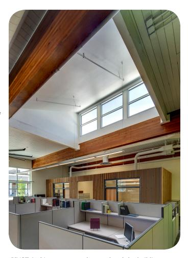
PIVOT Architecture recently completed the building remodel for Lane County's Public Works Customer Service Center, in which existing materials were re-purposed. Wood slat wall finish around new offices featured above were faced with salvaged decking material taken from the existing roof structure.
