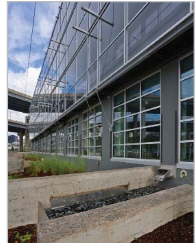
solar wall and stormwater feature
