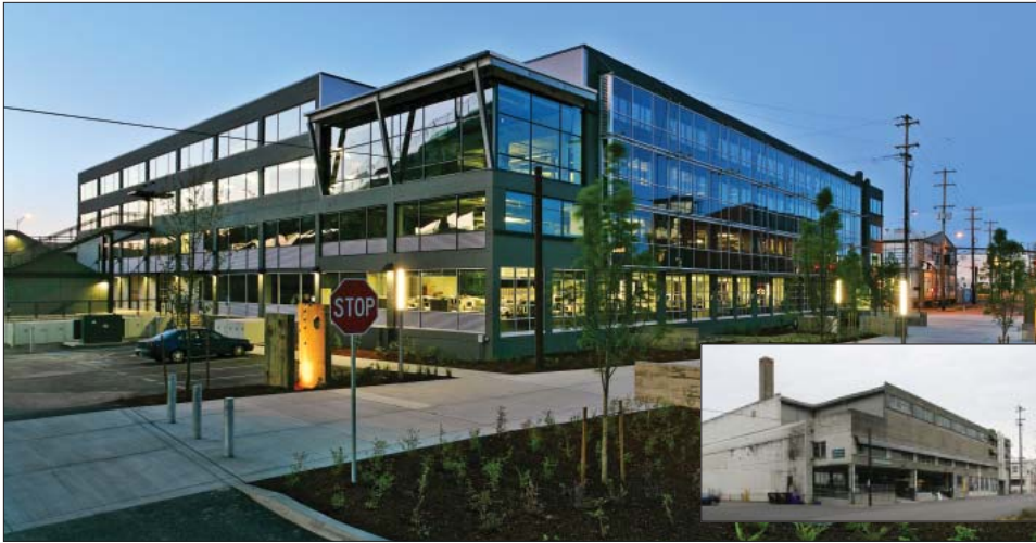
RiverEast Center, Portland, Ore.
