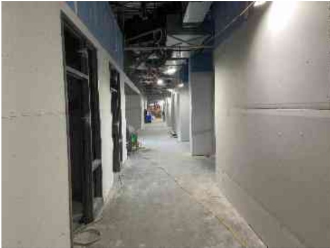
Drywall Application in Hallways
