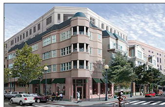
Bay Area Rapid Transit Parking Garage Walnut Creek, California
