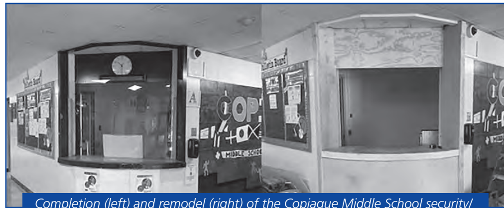
Completion (left) and remodel (right) of the Copiague Middle School security/greeter's entrance.
