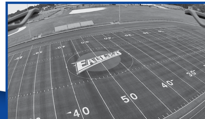
A new synthetic turf athletic field has been completed at Walter G. O'Connell Copiague High School.
