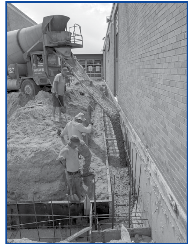
Concrete was poured for the Walter G. O'Connell Copiague High School addition, which will be renovated during the summer break in 2018. Heating and cooling work was also completed in the locker rooms.
