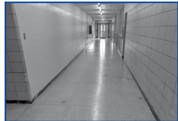
New terrazzo floors were installed during the summer at Copiague Middle School. Other work included new piping and ductwork outside the chorus room as well as renovations to the science rooms.
