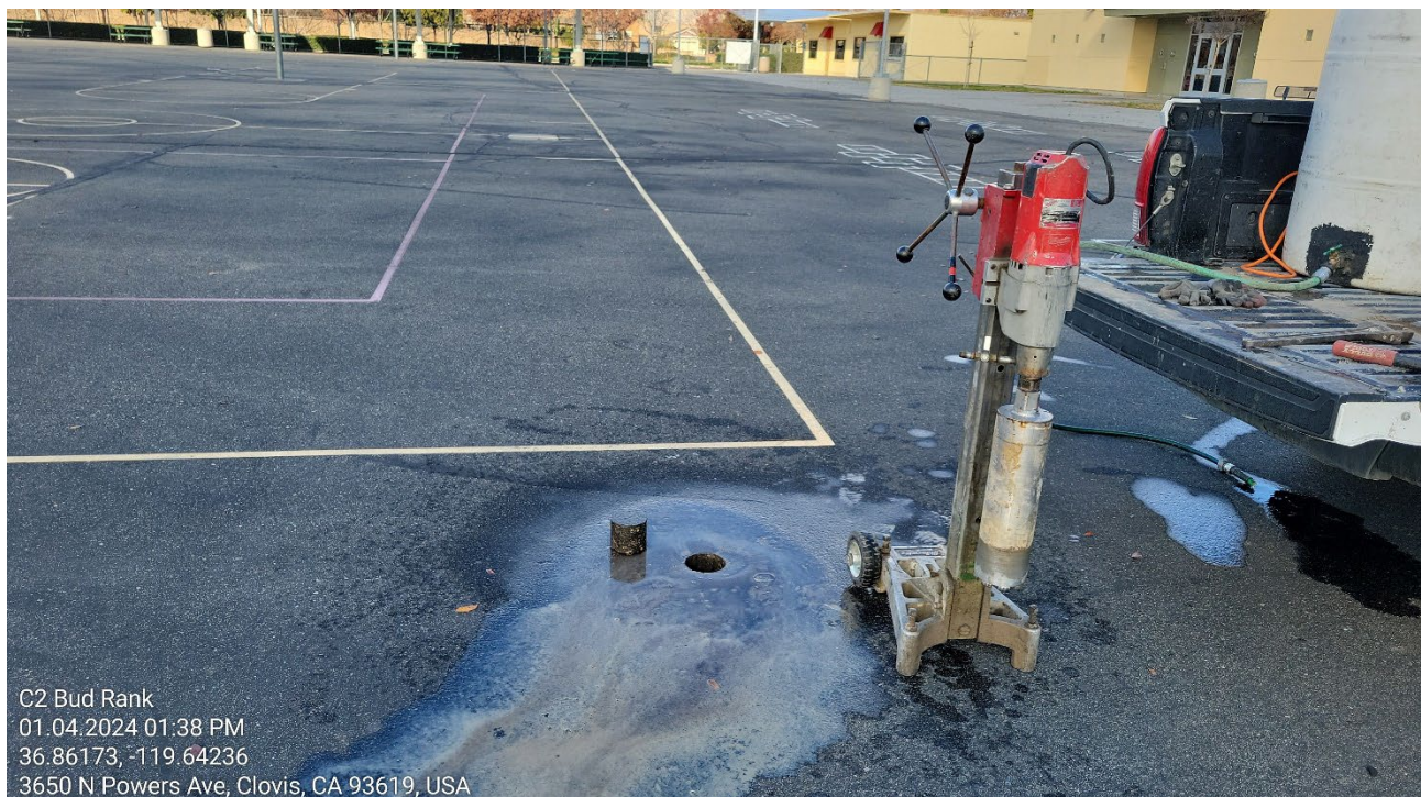
Photo taken from the southeast corner of the site (near C-2), facing north. Taken on January 4, 2023.
