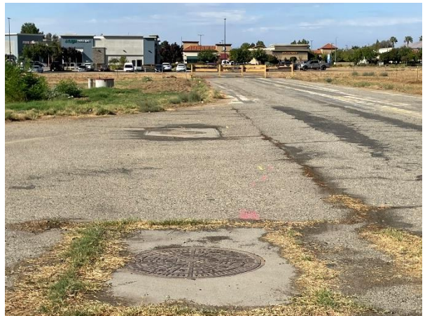
Photo 4. Old Alignment of N. Fowler Avenue. Facing North
