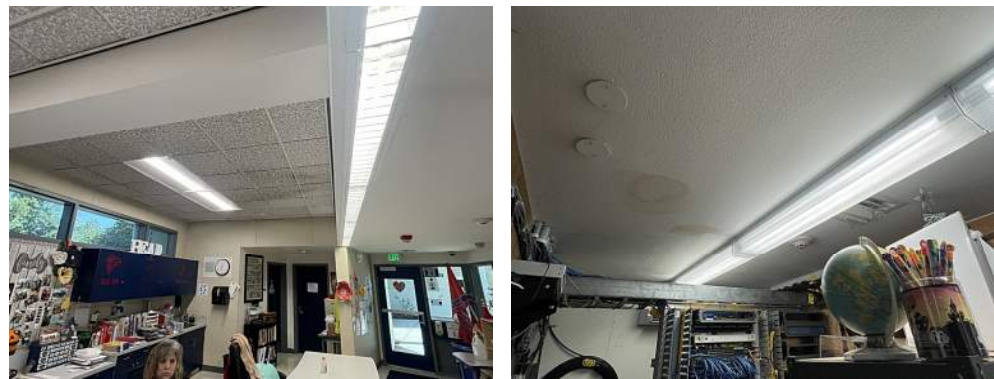
01 OVERALL PHOTOS OF LIBRARY AREAS
