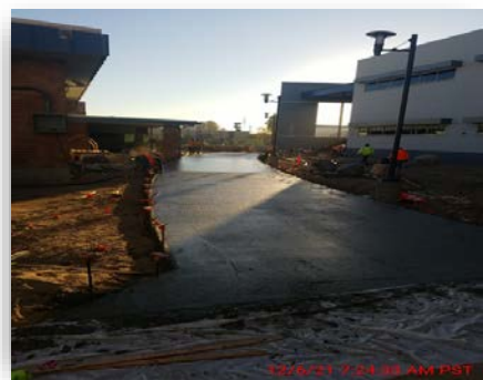
Figure #4 – Place Concrete @ NE Area of STEM December 6, 2021
