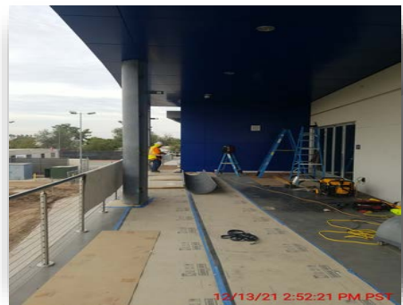
Figure #12 – Placement of GFRP Column Wraps December 13, 2021
