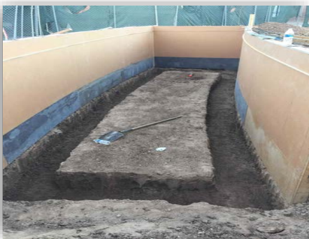
Figure #3 – Forming Planter Walls @ North Amphitheater December 2, 2021
