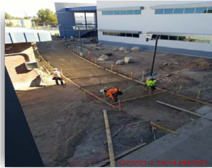
Figure #2 – Forming NE Hardscape Pathway December 2, 2021
