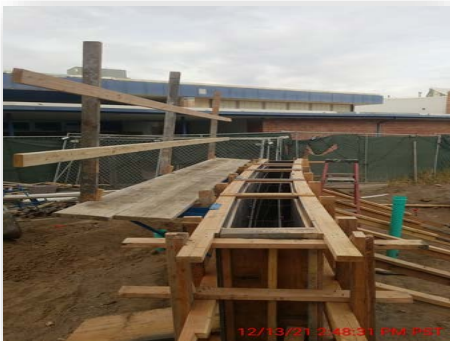
Figure #11 – Form Work @ NE Area of Stem December 13, 2021
