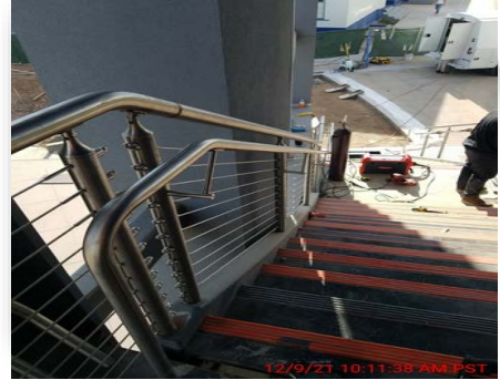
Figure #8 – Handrails @ East Main Entry Stairs December 9, 2021
