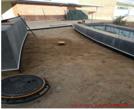
Figure #19 – Adjust & Set Time Capsule Cover to Grade December 27, 2021
