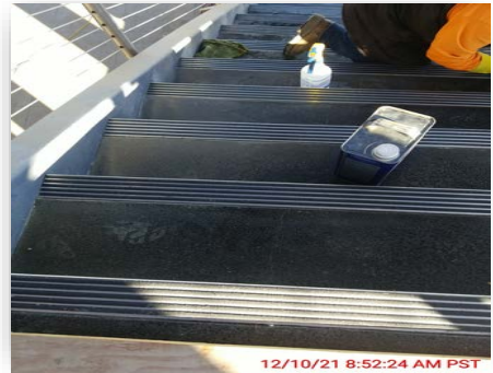
Figure #10 – Cleaning Up Stair Tread Nosing @ All Stairs December 10, 2021
