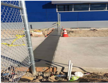
Figure #21 – Placed Concrete @ West Fence Area December 28, 2021
