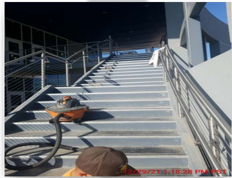
Figure #22 – Cleaning Stair Nose Treads @ East Stairs December 29, 2021
