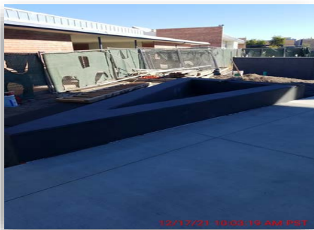
Figure #15 – Blasting Concrete Surfaces @ the NE Area December 17, 2021
