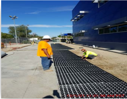
Figure #1 – Placing Gravel Pave Along Fire Lane December 1, 2021
