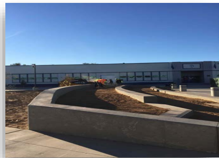
Figure #16 – Grading East Amphitheater Bench Area December 20, 2021
