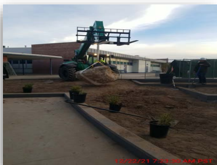
Figure #17 – Placement of Landscape DG @ Southeast December 22, 2021
