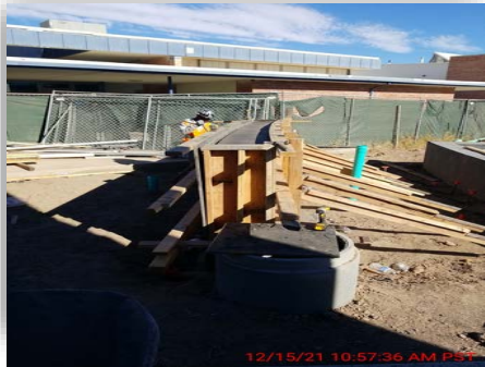
Figure #13 – Stripping Concrete Forms @ the NE Area December 15, 2021
