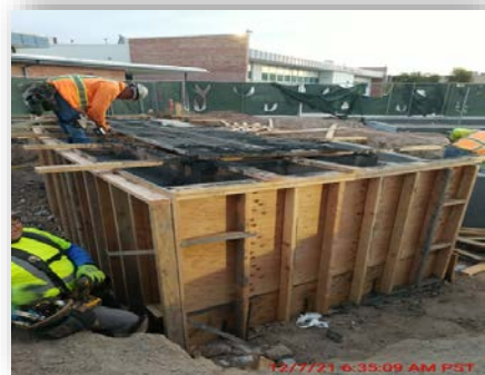
Figure #6 – Removing Forms From Planter @ NE December 7, 2021
