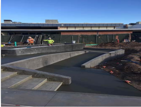
Figure #7 – Placing Concrete @ Ramp & Walkway Ribbons December 8, 2021
