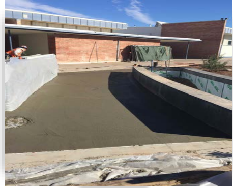
Figure #20 – Placed Concrete Flatwork @ NE Area December 28, 2021
