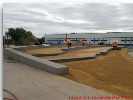
Figure #18 – Continue With DG Placement @ Southeast Area December 23, 2021
