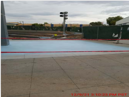
Figure #9 – Placing Concrete @ Hardscape Color Infills December 9, 2021
