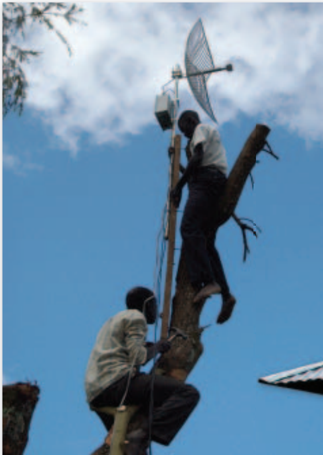
IT TAKES A VILLAGE Local residents carried equipment to Nyarukamba in the foothills of Uganda's Rwenzori mountains (top) and helped set up the solar panel that powers the village's wireless Internet system (right). An old tree trunk is being used as a mounting pole for the network's antenna (above).
