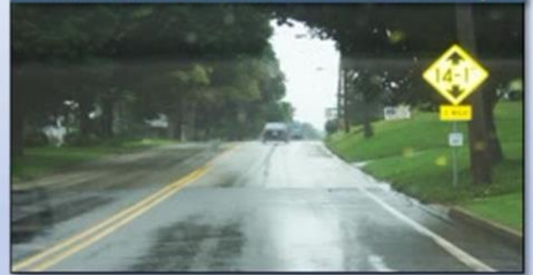
Water on the roadway
