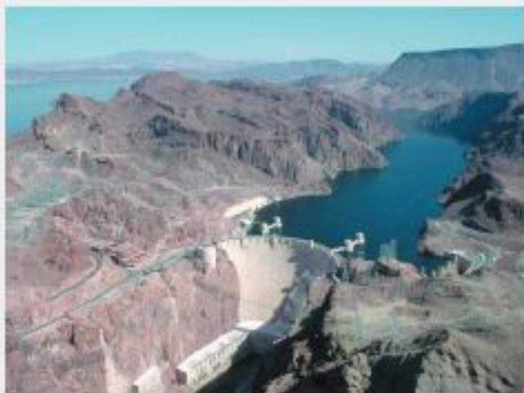
Lake Mead, behind the Hoover Dam, stores water for the people of the Southwest region.
