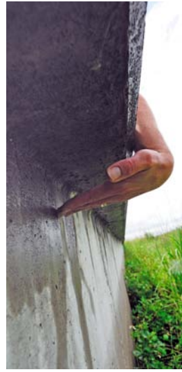
The lip along the top of this wall in Florida keeps small animals off the road (right), while the passage underneath (main) allows them to cross.
