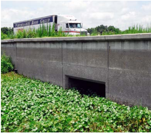
The lip along the top of this wall in Florida keeps small animals off the road (right), while the passage underneath (main) allows them to cross.
