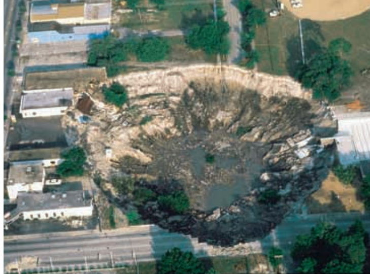
Figure 7 The damage to this city block shows the effects of a sinkhole in Winter Park, Florida.
