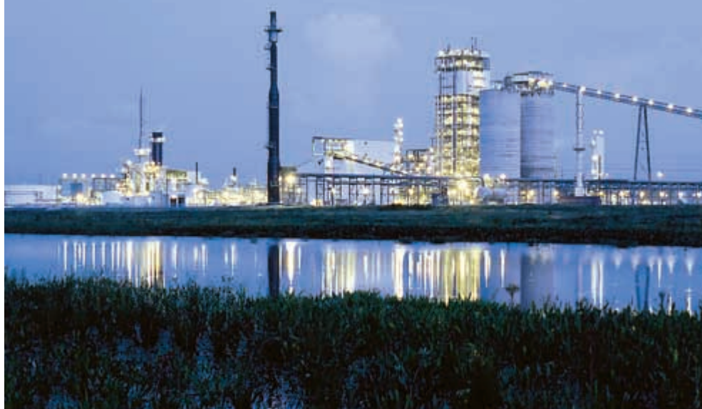
Figure 2 This power plant is leading the way in clean-coal technology. The plant turns coal into a gas before it is burned, so fewer pollutants are released.
