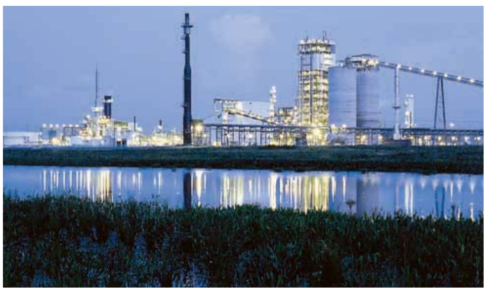
Figure 2 This power plant is leading the way in clean-coal technology. The plant turns coal into a gas before it is burned, so fewer pollutants are released.
