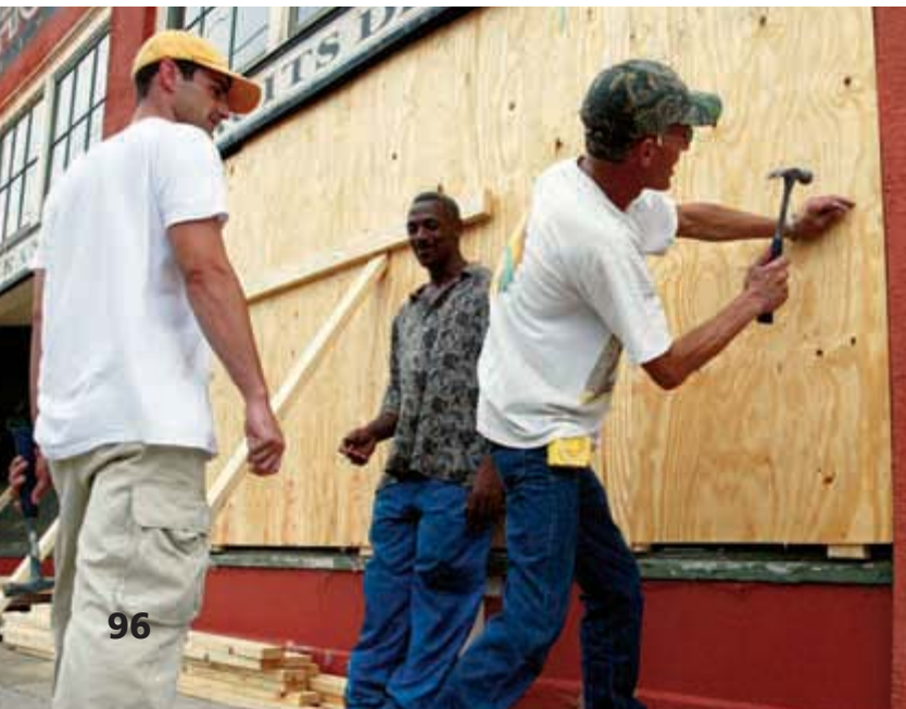
Figure 11 These store owners are boarding up their windows to protect the windows from strong winds during a hurricane.
