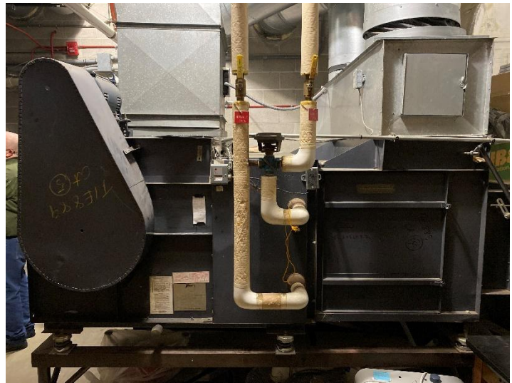
Boiler B-2 (Left) Air Handling Unit (Right)
