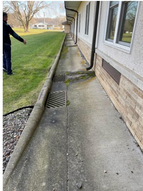
Mold Growth and Water Damage in Concrete Channel
