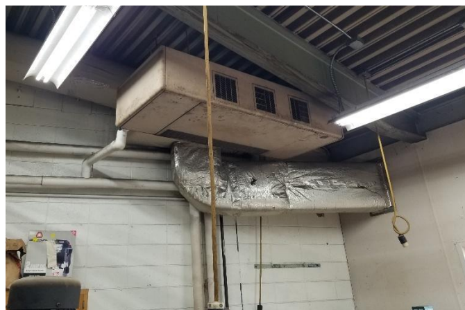
Air Handling Unit (Top Right) Unit Ventilator (Top Right) Exhaust Fan (Bottom Center)
