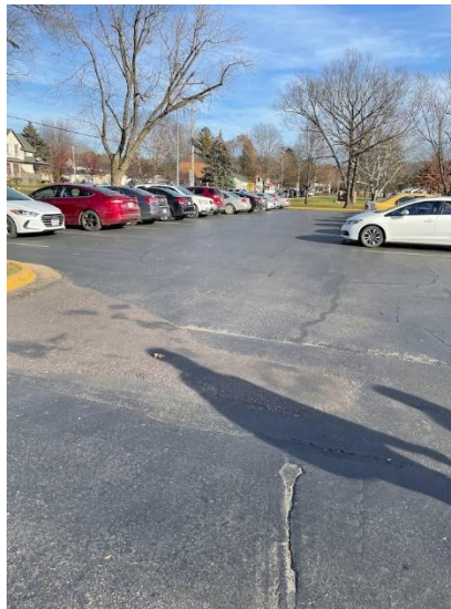
ADA Parking Areas (Left) and Asphalt Cracks (Center and Right)
