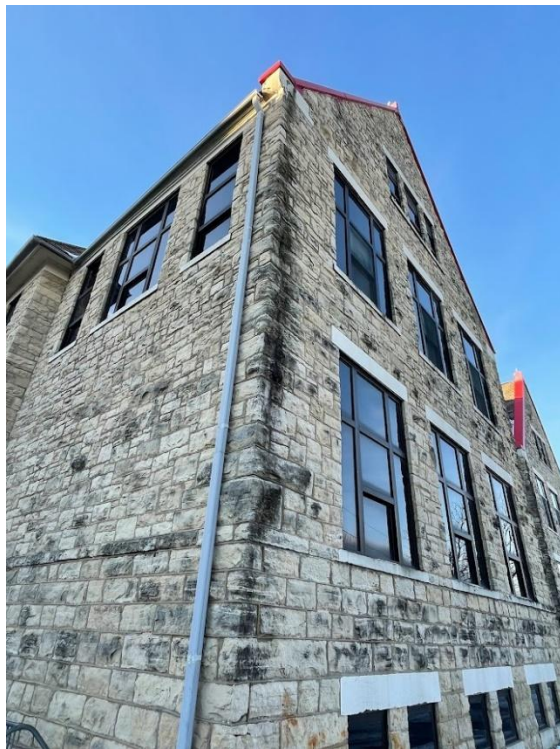
Damage and Staining to Stone Exterior
