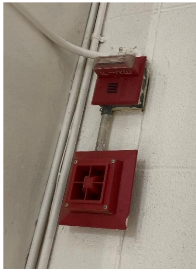
Existing Horn, Strobe and Pull Devices
