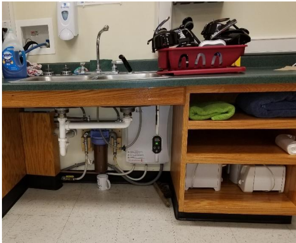
Below Sink Filter (Left) and Filter Behind Drinking Fountain ( Right)
